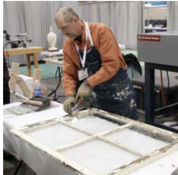
At one of the conference's demonstrations, contractor Marc Bagala shows how easily paint and glazing compound peel off a window sash that's spent a few minutes inside his invention, the Steam Stripper (partly visible at right).
