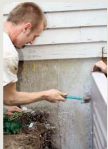
Figure 5. The ScapeWel sides should be placed at least 4 inches above grade to prevent debris (and people) from falling inside. The sides are fastened to the foundation with 1/4-inch wedge anchors. The flange can also be mounted directly to a metal window buck; it contains two hole patterns for different brands of basement windows.
