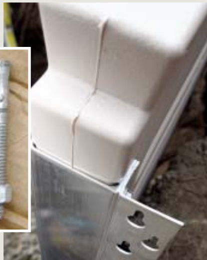
Figure 5. The ScapeWel sides should be placed at least 4 inches above grade to prevent debris (and people) from falling inside. The sides are fastened to the foundation with 1/4-inch wedge anchors. The flange can also be mounted directly to a metal window buck; it contains two hole patterns for different brands of basement windows.
