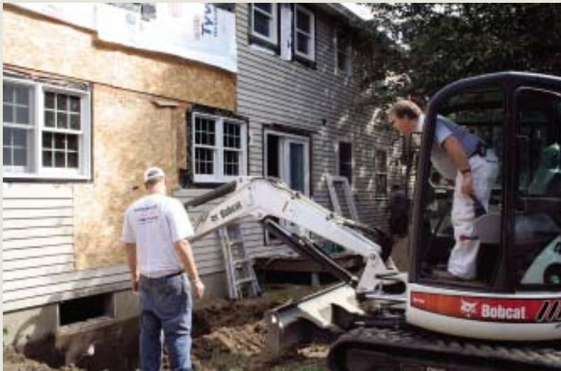
Figure 1. A second pair of eyes helps prevent the excavator from damaging underground utilities. The worker also provides hand signals so the operator can get the last few bucketfuls of loose soil out of the hole.
