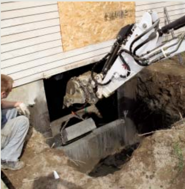
Figure 3. Cutting the 4-foot-square chunk of concrete into four pieces makes it easier to handle. One piece fell inside the basement; it was lifted out with a chain attached to the excavator's bucket.
