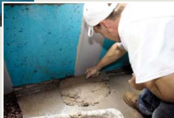
Figure 8. Installed at the base of the well, T-shaped drains (inset) prevent water from accumulating in the bottom of the well. They're run through holes in the foundation and dump water into 1/2-inch-thick flat piping on the inside of the foundation wall (above). More commonly used to collect seepage from foundation cracks, the flat piping is easier than conventional pipe to hide behind furred walls; it channels water into a foundation drain located under the basement slab. Once the pipe is routed into the drain, the floor is patched with sand mix (right).
