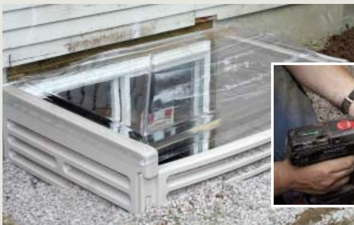
Figure 9. A clear plastic cover prevents debris and animals from getting inside the ScapeWel. Metal clips keep it in place in high winds but allow it to be easily opened from inside. For greater protection, a grated steel cover is available.
