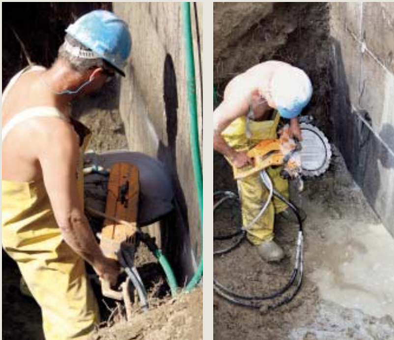
Figure 2. Powered by a portable gas-powered pump, a hydraulic cutoff saw provides smooth power without choking the operator with exhaust fumes. The operator first uses a cutoff saw, then switches to a ring saw to finish the cut. Both saws require a water supply (provided by a garden hose) to cool the blade and cut down on dust.
