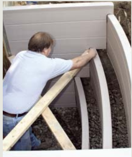
Figure 7. The manufacturer requires that the ScapeWel be backfilled with gravel; this reduces soil pressure that could distort the molded plastic. Prior to backfilling, the unit must be braced with 2x4s or 2x6s to prevent distortion.
