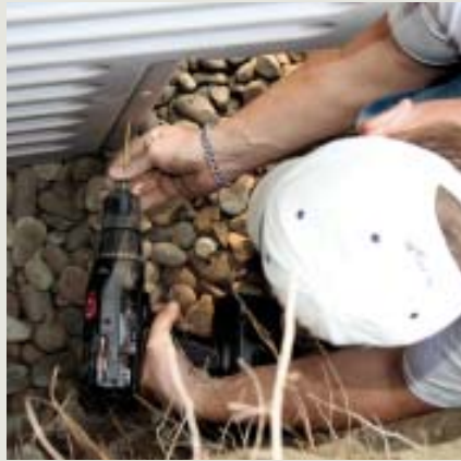
Figure 6. Before securing the step panels, workers check that the unit is square by taking diagonal measurements. Then they secure step panels to each side with a pair of 2½-inch coated deck screws.
