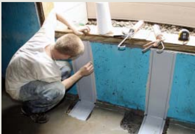
Figure 8. Installed at the base of the well, T-shaped drains (inset) prevent water from accumulating in the bottom of the well. They're run through holes in the foundation and dump water into 1/2-inch-thick flat piping on the inside of the foundation wall (above). More commonly used to collect seepage from foundation cracks, the flat piping is easier than conventional pipe to hide behind furred walls; it channels water into a foundation drain located under the basement slab. Once the pipe is routed into the drain, the floor is patched with sand mix (right).
