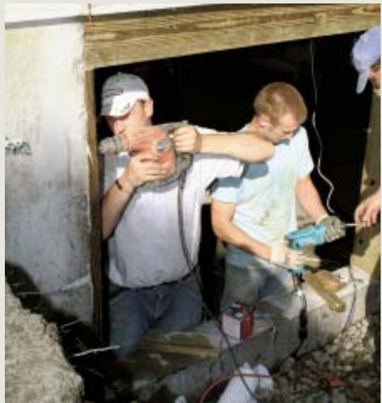
Figure 4. Concrete screws and a heavy dose of urethane construction adhesive are used to fasten the jack studs to the opening. Cutting the jack studs a little long and beating them into place ensured the header was carrying the load from above.
