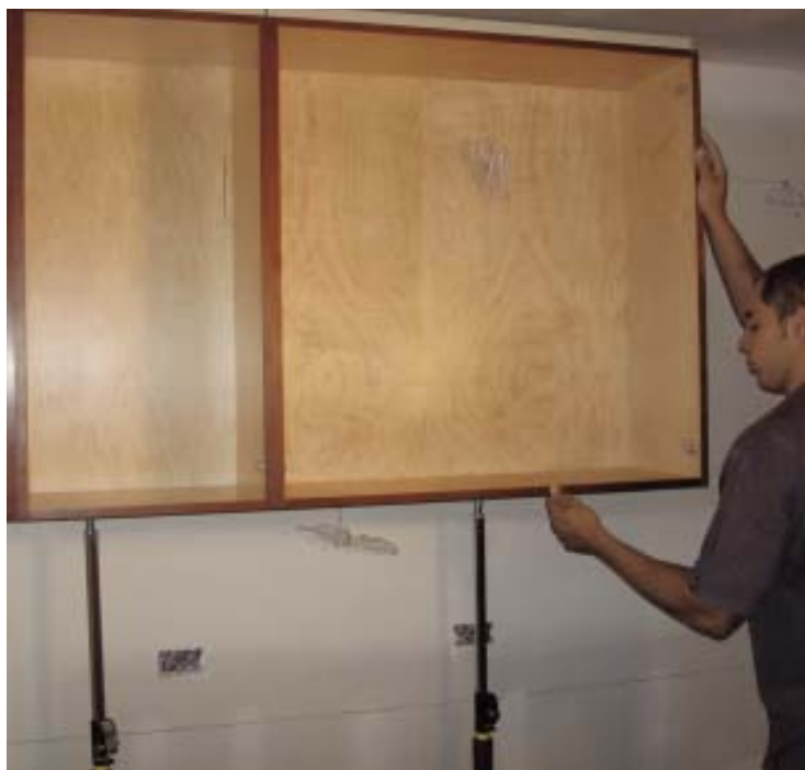
Essential tools for efficient cabinet installation include an assortment of drills and drivers, Pony Cabinet Claw clamps (top), and telescoping support poles (above).
