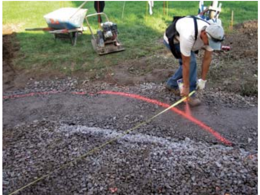
Figure 3. To prepare the site and prevent settling, the author stabilizes any loose fill, excavates about 8 inches below finish grade, and then builds up a compacted, well-drained stone base (left). This patio design, which will feature a low retaining-wall border, is laid out on the stone base with spray paint (below).
