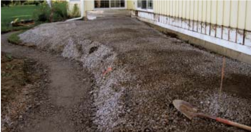
Figure 3. To prepare the site and prevent settling, the author stabilizes any loose fill, excavates about 8 inches below finish grade, and then builds up a compacted, well-drained stone base (left). This patio design, which will feature a low retaining-wall border, is laid out on the stone base with spray paint (below).
