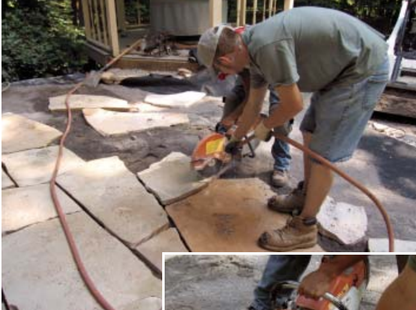
Figure 4. In some projects uncut flagstones are fit together loosely like a jigsaw puzzle; in this one, the stones are cut to fit, so that joints are tighter (above). With one stone overlapping another, the author's crew cuts through both stones at once (right), then finishes up by cleaning up the cut on the lower stone (below right).
