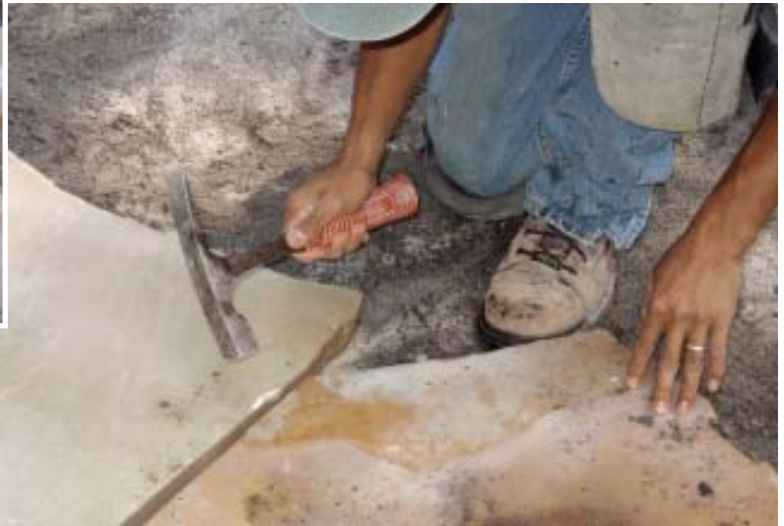
Figure 5. Because cut edges can look too symmetrical and matched (left), the author's crew chips them with brick hammers to give them a more natural look (below).
