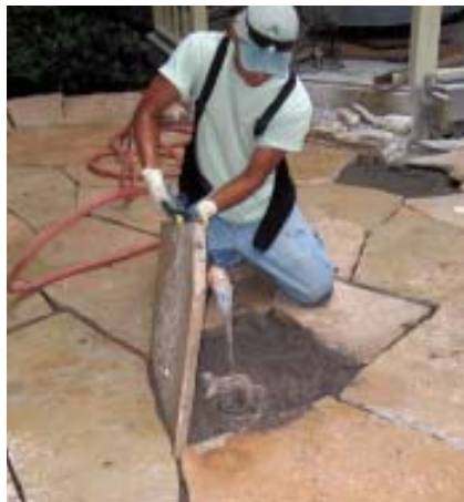
Figure 6. After the flagstones have been cut and fit together (left), the author's crew floods the concrete sand base underneath with water until it achieves a quicksand-like consistency (above left). Then the flagstones are set in place; a crew member wiggles each one and pushes wet sand out from between the joints to seat it fully (above right).
