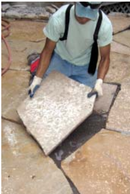
Figure 6. After the flagstones have been cut and fit together (left), the author's crew floods the concrete sand base underneath with water until it achieves a quicksand-like consistency (above left). Then the flagstones are set in place; a crew member wiggles each one and pushes wet sand out from between the joints to seat it fully (above right).
