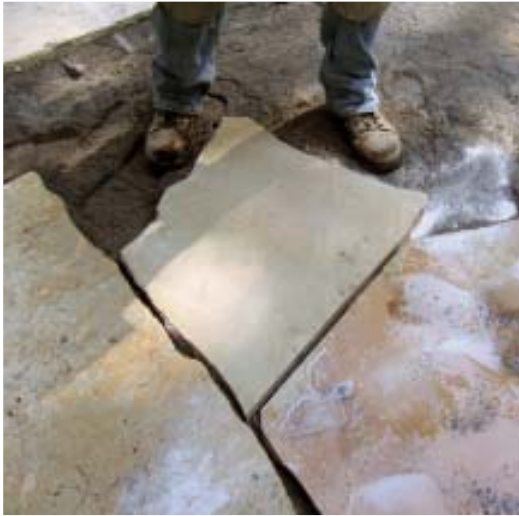
Figure 5. Because cut edges can look too symmetrical and matched (left), the author's crew chips them with brick hammers to give them a more natural look (below).
