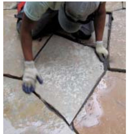
Figure 6. After the flagstones have been cut and fit together (left), the author's crew floods the concrete sand base underneath with water until it achieves a quicksand-like consistency (above left). Then the flagstones are set in place; a crew member wiggles each one and pushes wet sand out from between the joints to seat it fully (above right).
