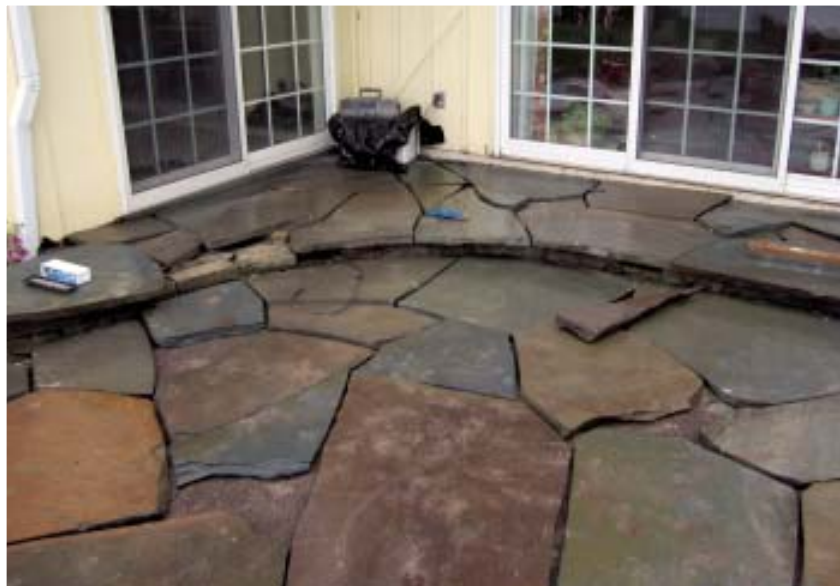
Figure 7. Once the stones are seated and the patio surface is level (left), polymer sand is swept into the joints, which locks the stones in place and minimizes weed growth (below).
