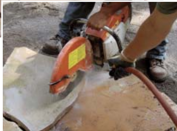
Figure 4. In some projects uncut flagstones are fit together loosely like a jigsaw puzzle; in this one, the stones are cut to fit, so that joints are tighter (above). With one stone overlapping another, the author's crew cuts through both stones at once (right), then finishes up by cleaning up the cut on the lower stone (below right).
