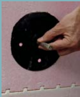
Figure 2. Plan ahead to attach to ICFs. A plastic anchor tunnel screws into a hole drilled in the ICF. The tunnel holds an anchor bolt square to the wall, and the concrete is poured around it. Tunnels are installed in a staggered line to minimize forces that might split the ledger.
