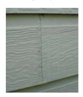
sort — it's at the bottom of the butt joint in the siding. I'd like to know what this is. We've been having problems with buckling of fiber-cement siding, and I wonder if the clips might provide a more secure attachment.
