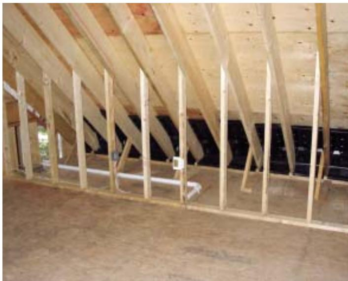
a top plate, which eliminates the twisting in the studs and helps to distribute the flexing that rafters are prone to. Before building the knee wall, I first insulate the rafters with fiberglass, then install a poly vapor retarder before attaching the knee-wall top plate.
