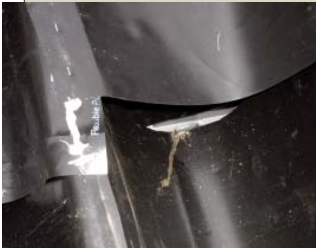
Figure 12. Just a slit between the troughs and the baffle shows water's path into the gutter below. There are a couple of inches of clearance between the main trough and the return to prevent debris from hanging up and clogging.
