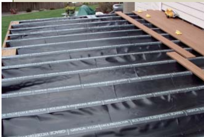
Figure 10. Grace Deck Protector caps the joists and the polypropylene membrane, adding a layer of protection that self-seals around the decking screws. Note the Deck Protector continuing up the wall, lapping the joint between the pieces of membrane.
