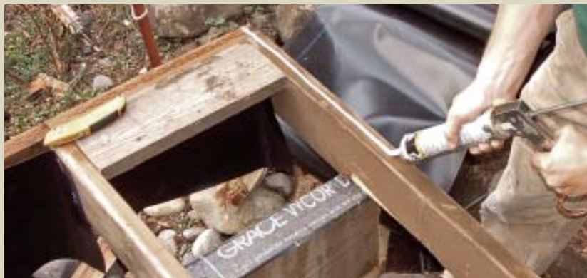
Figure 6. Polyurethane caulk seals the membrane to the joists.
