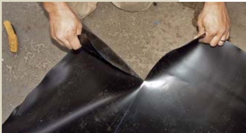
Figure 4. After the polypropylene membrane is laid out on a concrete slab and scored with a utility knife, the membrane tears easily. It's best not to cut all the way through, to preserve the knife's sharpness.
