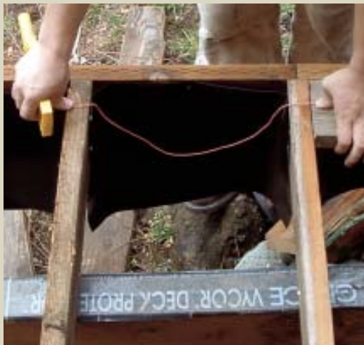
Figure 2. Use a string to measure the span of the membrane. On the gutter end, it should droop almost to the bottom of the joists. On the house end, it should droop down only an inch or so.
