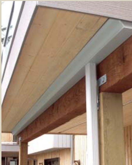
Figure 5. Traditional aluminum or plastic gutter affixed to the main beam carries away the water from the membrane troughs.
