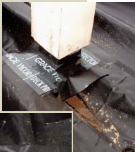
Figure 14. To waterproof around details such as posts (right) and steps (below), the author stacks the layers with the upper over the lower, just like roofing, and uses Deck Protector as flashing.
