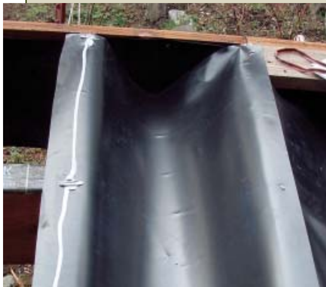
Figure 9. A bead of caulk atop the first piece of membrane seals the joint. Be sure to caulk over the staples to prevent leaks.
