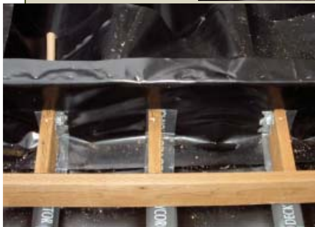
Figure 14. To waterproof around details such as posts (right) and steps (below), the author stacks the layers with the upper over the lower, just like roofing, and uses Deck Protector as flashing.
