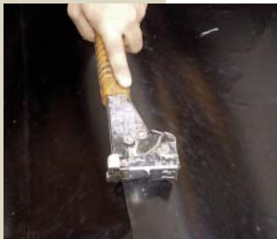
Figure 8. A stapler is used both to attach the membrane and to smooth out the caulk under the layers of membrane.
