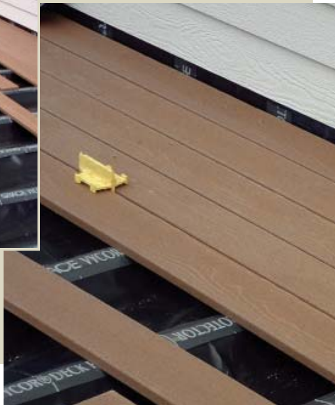
Figure 10. Grace Deck Protector caps the joists and the polypropylene membrane, adding a layer of protection that self-seals around the decking screws. Note the Deck Protector continuing up the wall, lapping the joint between the pieces of membrane.
