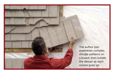
To simplify pattern orientation during layout and shingle installation, I snap two exposure course lines across each group of shingles that constitutes a course. I match the lines to the story pole so the exposures correspond to the courses on the wall, and I use white chalk, which can easily be brushed away if needed.
