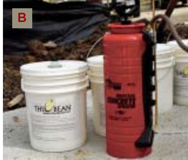
Figure 5. To slow hydration, newly placed pervious concrete is sprayed with a soybean-based curing compound (A, B), then quickly covered with polyethylene sheeting (C). The sheeting is weighted down with sandbags and left in place for seven days (D), and the paving is allowed to fully cure for 21 days before being opened up to vehicle traffic.
