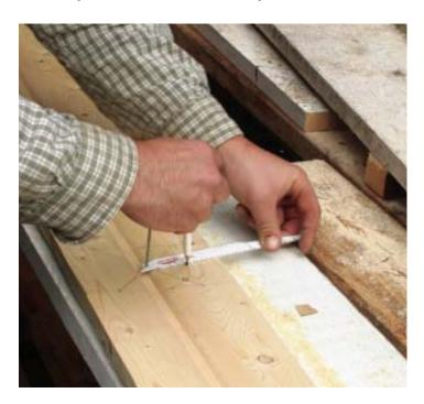
hen installing siding or soffits, you frequently have to cut circular openings for pipes, vents, and electrical boxes.
