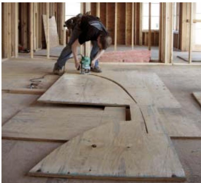
flush-cutting the sheathing at the perimeters of walls, and routing off the excess ply at the edges of floors. Marking and cutting the floor sheathing at a bay window takes time; running the sheathing long and cutting it flush with a router is quicker and more precise (1). A nice thing about routing the edge of a deck is you can hook your tape there to pull dimensions and know you're measuring from the face of the rim.
