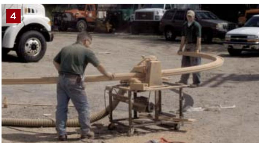
The gutter slopes back toward the house and drains to a pair of downspouts. Once installed, it was finished in the traditional New England manner: The outside was painted and the inside was coated with linseed oil. Since mahogany is naturally rot-resistant, the gutter will be durable even if the homeowner forgets to periodically renew the linseed-oil coating. — *David Frane*
