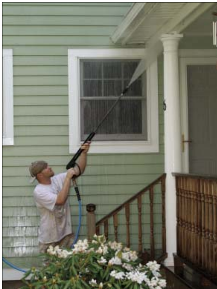
A thorough and vigorous washing is the best prep for routine repainting. Don't neglect the areas under eaves — they can accumulate salt and grime deposited by moisture rising up from soil around the building.
