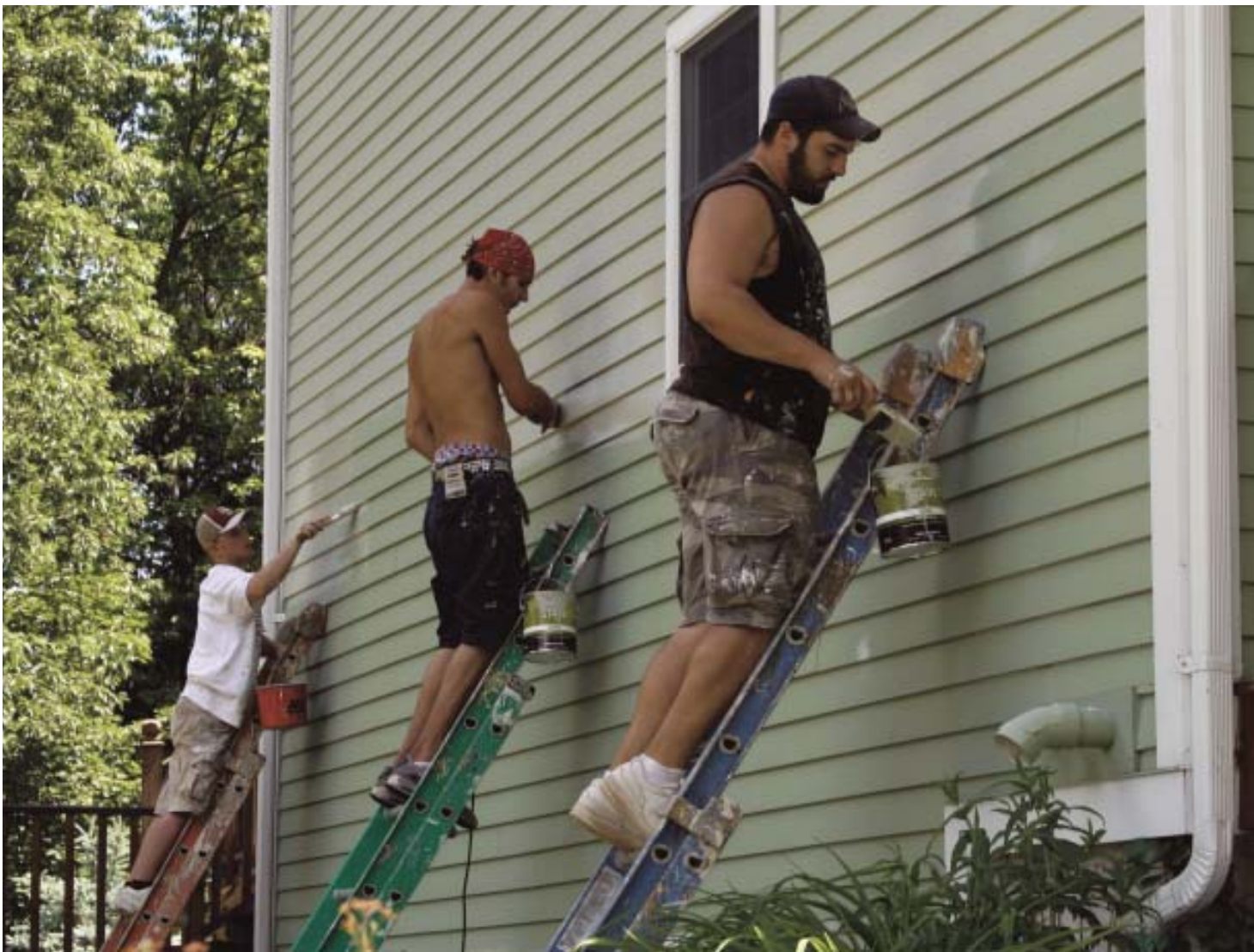
Three painters work together on the shady side of a house to get the paint on quickly. Modern acrylic paints and stains tend to dry quickly compared with older, higher-VOC formulas.
