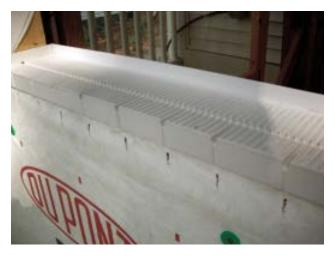
Missing-Pan Plan. Short of removing the entire unit, what are your options when you come across a leaky window with no pan installed? According to its maker, the *DamSill Window Pan* can be installed under existing windows and doors. The technique was perfected on leaky SIPs buildings as part of a class-action lawsuit settlement. Videos on the manufacturer's Web site demonstrate both new and retrofit installations. The pans sell for \$11 each with a 200-count order.
