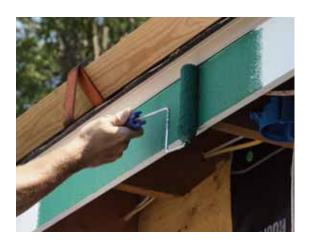
Paint It Black. Makers of cellular PVC exterior trim warn that painting their products dark colors can intensify the effects of expansion and contraction and lead to warping. However, Sherwin-Williams says its new *VinylSafe* paint has no such effect: According to the company, all 100 shades reflect light so effectively they can be applied to cellular PVC with no risk of warping. The paint costs \$39 for flat, \$42 for satin, and \$43 for gloss.
