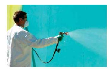
Farewell, Fasteners. In areas where driving rain is an issue, fastener holes can be a source of moisture penetration. Grace has a solution: Its *Perm-A-Barrier VP* membrane goes on as a spray, no fasteners needed. The acrylic fluid cures into a vapor-permeable monolithic sheet that keeps out liquid water. A 5-gallon container sells for \$135, a 55-gallon drum for \$1,350.
