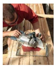
When rafters are gang cut, the saw's cutting capacity helps determine birdsmouth dimensions: a 10<sup>1</sup>/4-inch Big Foot saw is capable of making a 3-inch seat cut, which is suitable for a wide range of roof pitches and rafter sizes.
