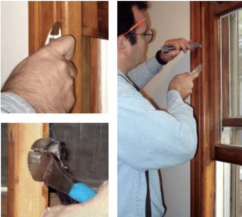
Figure 4. After scoring the joints with a sharp utility knife, the author inserts a putty knife and a thin pry bar between the interior stop and the jamb, then carefully pries away the stop. Since these stops will be reinstalled later, they have to be removed carefully.
