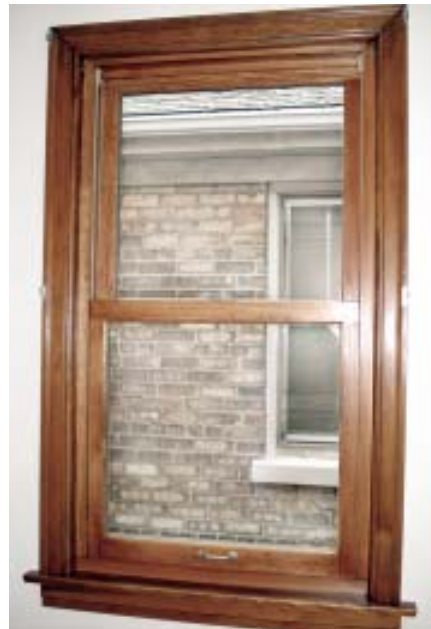
Figure 11. The last step is reinstalling the stops. The author fastens them with a Paslode cordless brad nailer, which spares him from having to drag a potentially dirty and dangerous air hose through the client's home. Once the new window is finished, it looks very similar to the original — except it's more energy-efficient and tilts in for cleaning.
