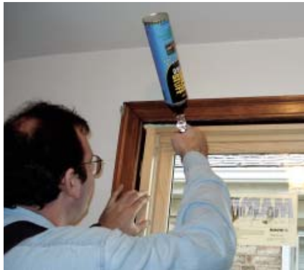
Figure 10. Polyurethane-foam window and door insulation fills the gap between the new window and the old opening. A high-quality professional foam gun provides greater control and makes less mess than straw-equipped cans.
