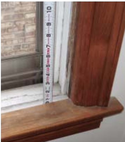
Figure 1. It's important to measure both the width and the height of the sash opening in at least three places, then use the smallest measurement for ordering. The ideal way to measure for height is to open both sash and slide a tape measure between them, but if the top sash is painted shut, the author measures from the head jamb to the bottom of the stool.
