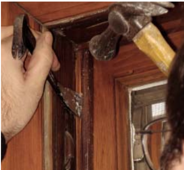
Figure 5. Less care is required when removing parting stops, which won't be reused. A pair of locking pliers provides a good grip, making it easier to pop out the smooth-sided stop.
