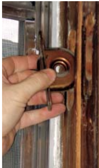
Figure 6. Weight pockets are located on the side jambs, behind rabbeted doors typically secured with flat-head wood screws. Once the doors are removed, the weights and pulleys can be taken out and discarded.
