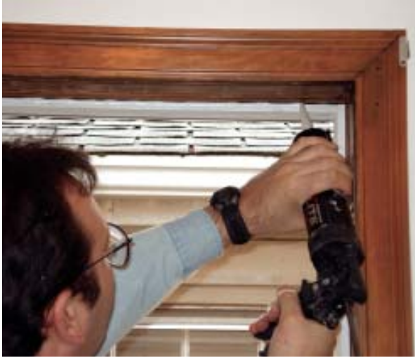
Figure 8. The author sets the new window against the outer stop in a bed of butyl caulk. Butyl sticks well to both aluminum and old wood, and its non-hardening formula helps it absorb seasonal movement better than other sealants.
