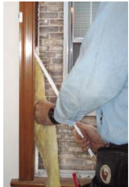
Figure 7. After the old balance system has been removed, the weight pockets are filled with fiberglass. To confirm that the insulation has reached the top of the pocket, the author looks into the hole that previously housed the sash weight pulley.
