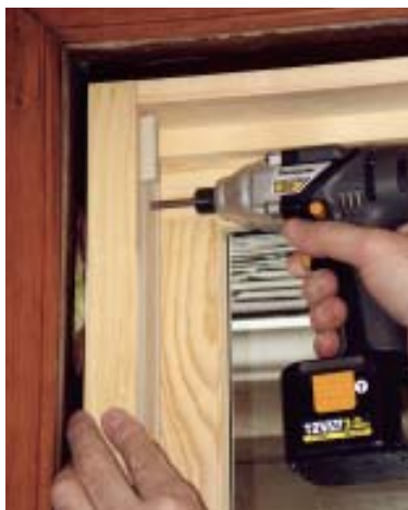
Figure 9. With screws, the author secures the new window in the opening. The center “jack” screw adjusts the reveal for the best appearance and smooth operation. Plugs hide the screws on the interior and exterior; a piece of weather stripping hides the jack screw.
