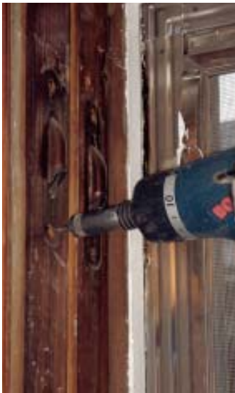
Figure 6. Weight pockets are located on the side jambs, behind rabbeted doors typically secured with flat-head wood screws. Once the doors are removed, the weights and pulleys can be taken out and discarded.
