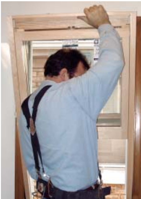
Figure 9. With screws, the author secures the new window in the opening. The center “jack” screw adjusts the reveal for the best appearance and smooth operation. Plugs hide the screws on the interior and exterior; a piece of weather stripping hides the jack screw.
