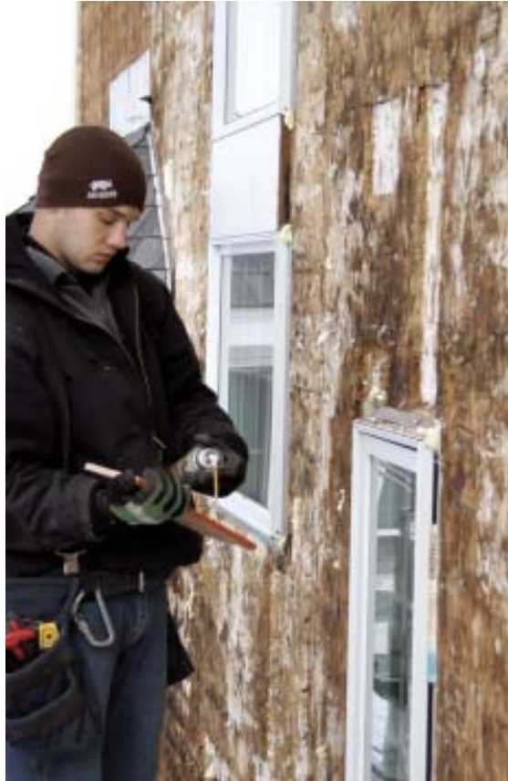
Figure 7. Heavily damaged sections of the SIPs panels were patched with OSB inserts secured with polyurethane foam.
