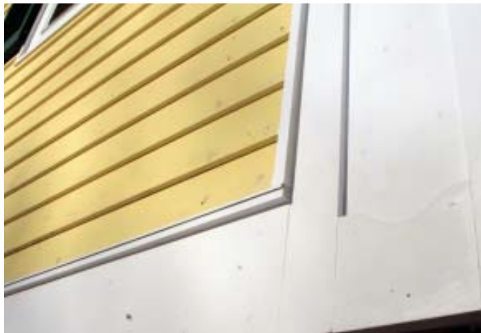
Figure 4. A 2-inch-wide backband applied to casings and corner boards made it possible to install the new clapboards over a \frac{3}{4} -inch air space without having to reset the windows.
