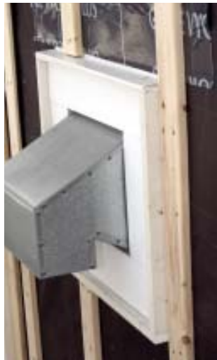
Figure 8. Spruce strapping over 30-pound felt provides a \frac{3}{4} -inch air space and drainage plane, so that the new clapboards can dry when wetted and infiltrating water can drain freely (left). Flashings were either tucked beneath the felt or sealed to the felt with Vycor (above left). Note the backband detail around the window trim (above right).
