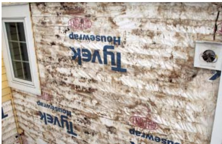
Figure 3. Brown stains from water-soluble extractives in the unprimed clapboards clearly indicate the movement of water. The damage was much worse on the southern exposure, where solar vapor drive played a role.
