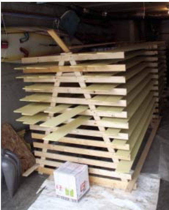
Figure 6. While the members of the mold remediation company did their work, the carpenters primed and painted the new clapboards in the garage (left), and replaced rotten trim, making sure to prime every cut (above).
