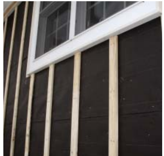
Figure 8. Spruce strapping over 30-pound felt provides a \frac{3}{4} -inch air space and drainage plane, so that the new clapboards can dry when wetted and infiltrating water can drain freely (left). Flashings were either tucked beneath the felt or sealed to the felt with Vycor (above left). Note the backband detail around the window trim (above right).
