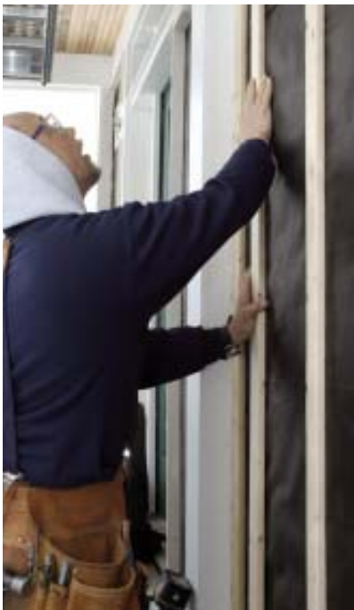
Figure 8. Spruce strapping over 30-pound felt provides a \frac{3}{4} -inch air space and drainage plane, so that the new clapboards can dry when wetted and infiltrating water can drain freely (left). Flashings were either tucked beneath the felt or sealed to the felt with Vycor (above left). Note the backband detail around the window trim (above right).
