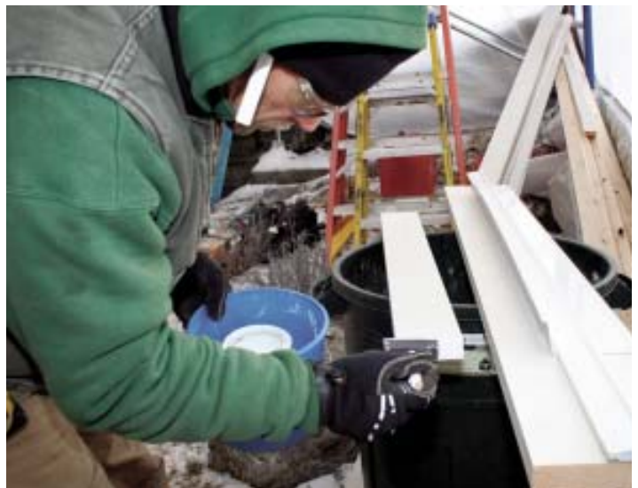
Figure 6. While the members of the mold remediation company did their work, the carpenters primed and painted the new clapboards in the garage (left), and replaced rotten trim, making sure to prime every cut (above).
