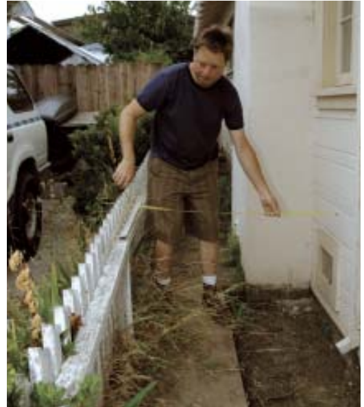
Figure 2. An electrician verifies that there will be the required 36 inches of clearance in front of the new panel within the property line.
