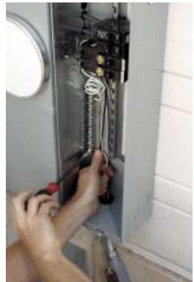
Figure 5. The electrician uses a rotary hammer with a ground-rod-driving attachment to drive a grounding rod into the soil (top left). He then runs a single grounding wire that connects to a clamp on the water main (top right), an acorn clamp on the ground rod (above left), a lay-in lug on the grounding bushing on the conduit to the loads (not shown), and the neutral bus in the main service (above right).
