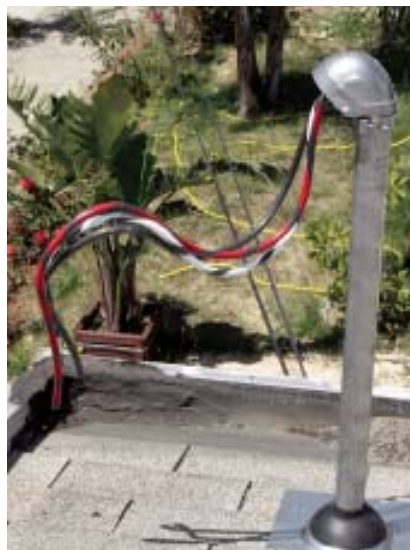
Figure 4. Gravity makes it easier to “pull” service conductors (left) by pushing them into the conduit from above. The electrician uses colored tape to color-code conductors so the utility knows which two to connect to the hots and which one to connect to the neutral (above left). Once the conductors are in the meter-main, the electrician connects the hots (red/black) to the line-side lugs, and the neutral (white) to a lug that ties to the neutral bus in the distribution section (above right).
