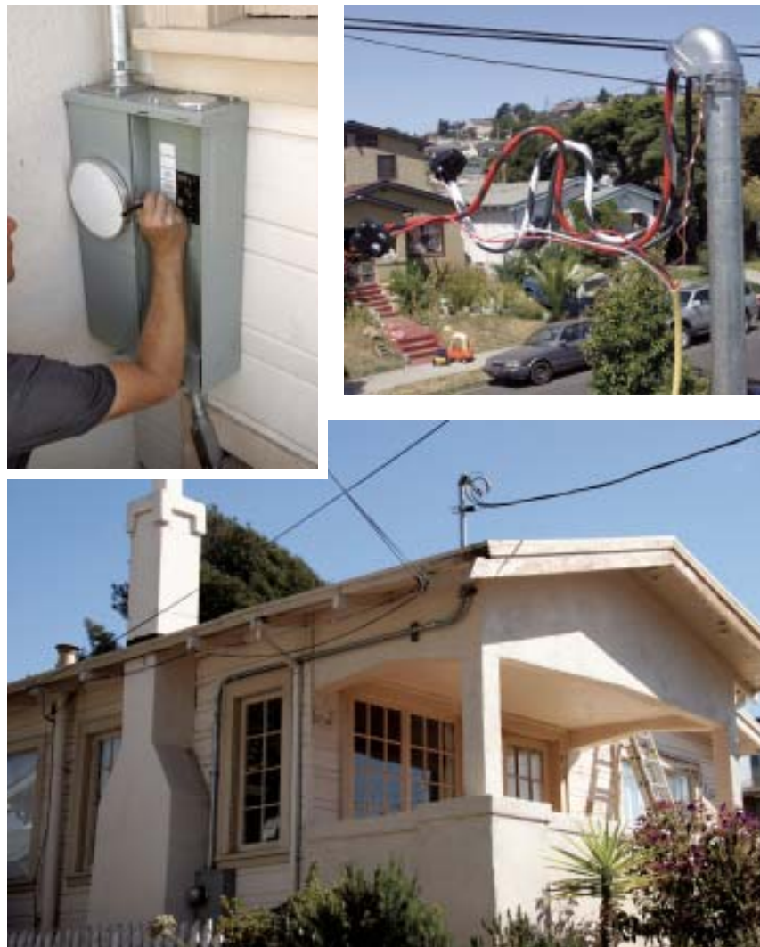
Figure 8. Once the loads have been transferred to the new panel, the electrician labels the circuits (top left) and installs the cover. Since the house was occupied and it was going to be some time before the utility could show up and make the final connection, the author's crew supplied temporary power by running Romex between the existing service drop and the new service conductors (top right). Later, the utility came out, removed the jumpers and existing service drop, and connected the new service drop (above).
