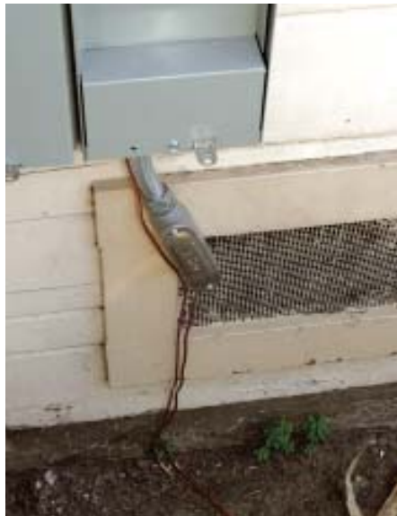
Figure 5. The electrician uses a rotary hammer with a ground-rod-driving attachment to drive a grounding rod into the soil (top left). He then runs a single grounding wire that connects to a clamp on the water main (top right), an acorn clamp on the ground rod (above left), a lay-in lug on the grounding bushing on the conduit to the loads (not shown), and the neutral bus in the main service (above right).
