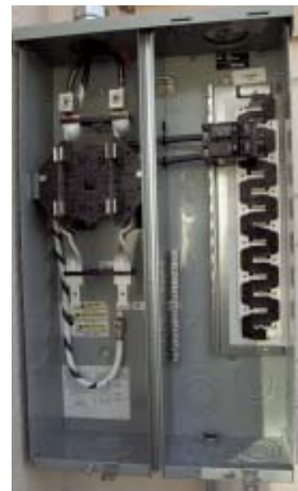
Figure 4. Gravity makes it easier to “pull” service conductors (left) by pushing them into the conduit from above. The electrician uses colored tape to color-code conductors so the utility knows which two to connect to the hots and which one to connect to the neutral (above left). Once the conductors are in the meter-main, the electrician connects the hots (red/black) to the line-side lugs, and the neutral (white) to a lug that ties to the neutral bus in the distribution section (above right).
