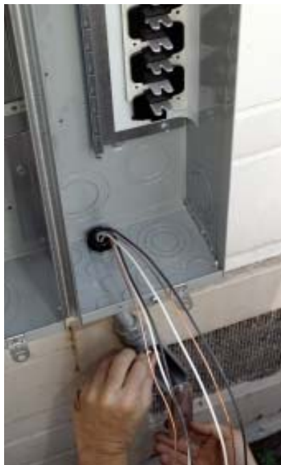
Figure 7. The electrician transfers the existing loads by disconnecting the knob-and-tube wiring from the fuse "panel" and running it to a junction box in the crawlspace, where it's connected to Romex (above). From there, the Romex runs to the other side of the house, exits the wall through a piece of conduit, and enters the bottom of the service panel (right).
