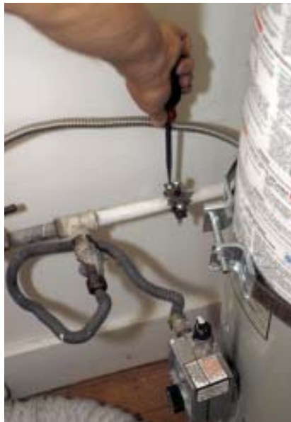
Figure 6. If the house has a gas line, the water pipes must be bonded to it. This is usually done at the water heater because both pipes are accessible there. A single length of grounding wire is connected to clamps on the water lines into and out of the heater (above left), then to a clamp on the gas line. The electrician installs a grounding clamp on the gas line (above right) after scraping off paint to ensure metal-to-metal contact.
