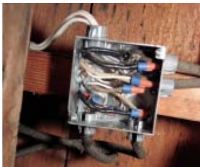
Figure 7. The electrician transfers the existing loads by disconnecting the knob-and-tube wiring from the fuse "panel" and running it to a junction box in the crawlspace, where it's connected to Romex (above). From there, the Romex runs to the other side of the house, exits the wall through a piece of conduit, and enters the bottom of the service panel (right).
