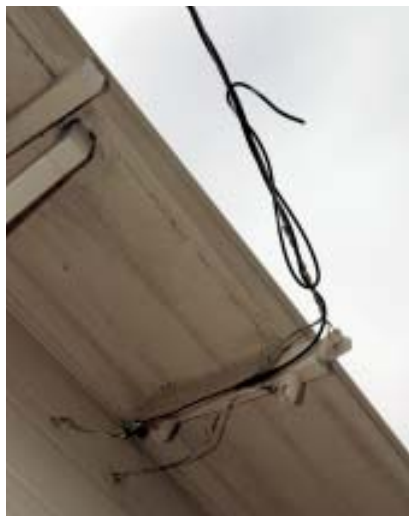
Figure 1. The author's company was hired to replace this original 1920s electrical service; it posed a hazard because it was old, undersized, not grounded, and in an outdoor ground-level wooden enclosure next to the driveway (above left). The service drop was connected to knob-and-tube wiring, which entered the building through holes in the wall. One of the hots was bent back and not connected (above right), so the house had only two-wire 120-volt service.
