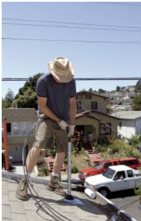
Figure 4. Gravity makes it easier to “pull” service conductors (left) by pushing them into the conduit from above. The electrician uses colored tape to color-code conductors so the utility knows which two to connect to the hots and which one to connect to the neutral (above left). Once the conductors are in the meter-main, the electrician connects the hots (red/black) to the line-side lugs, and the neutral (white) to a lug that ties to the neutral bus in the distribution section (above right).
