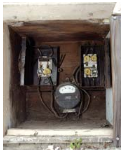
Figure 1. The author's company was hired to replace this original 1920s electrical service; it posed a hazard because it was old, undersized, not grounded, and in an outdoor ground-level wooden enclosure next to the driveway (above left). The service drop was connected to knob-and-tube wiring, which entered the building through holes in the wall. One of the hots was bent back and not connected (above right), so the house had only two-wire 120-volt service.
