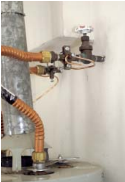
Figure 6. If the house has a gas line, the water pipes must be bonded to it. This is usually done at the water heater because both pipes are accessible there. A single length of grounding wire is connected to clamps on the water lines into and out of the heater (above left), then to a clamp on the gas line. The electrician installs a grounding clamp on the gas line (above right) after scraping off paint to ensure metal-to-metal contact.
