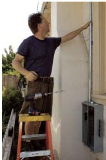
Figure 3. With the new meter-main firmly bolted to framing, the electrician installs a vertical section of the service conduit (above left). To avoid running the service drop over the neighbor's property, it was necessary to run the conduit to the front corner of the building before turning it up and passing it through the roof overhang (above right).
