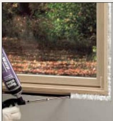
Some contractors try to air seal windows by stuffing fiberglass in the crack, but this won't work. Fiberglass doesn't stop air movement. A low-expanding foam sealant will.
