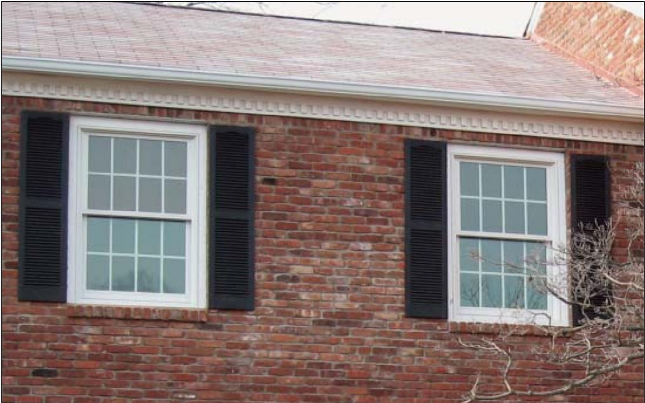
The key to a flawless window replacement in a brick-veneer wall is sizing the new window properly. The replacement unit must be small enough to fit through the existing brick opening without having to dismantle the brick and mortar, but large enough to minimize the unsupported flashing and allow the new unit to be inconspicuously trimmed out.
