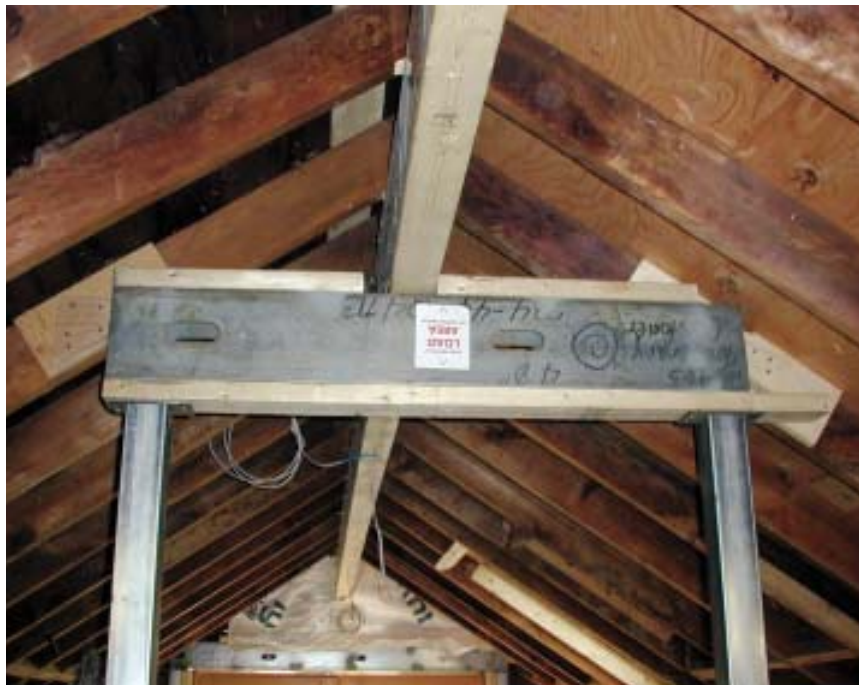
Figure 1. To keep the depth of the structural ridge to a minimum, the author chose Metwood TruSpan beams, which are made from cold-formed steel with internal reinforcing bar welded on for extra strength. The beams can be ordered with two-by nailers on top and bottom for fastening to wood framing.
