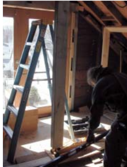
Figure 3. Temporary collars supported the chain hoist and ratchet straps (above left) used to lift the beams as high as possible, where they were supported from beneath with additional cross ties (above). A hydraulic jack (left) finished the job.
