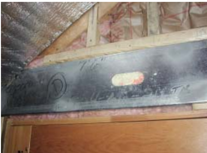
Figure 4. The Metwood headers for the gable walls came with punch-outs that allowed the author to insulate the cavities with spray foam.
