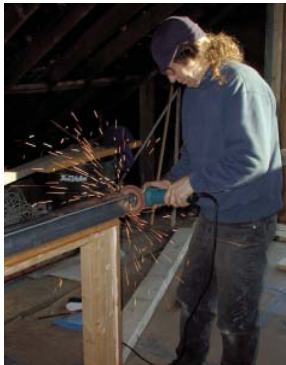
Figure 2. The Metwood beam can be cut easily with an abrasive blade on a chop saw (top) and trimmed with a grinder (above).
