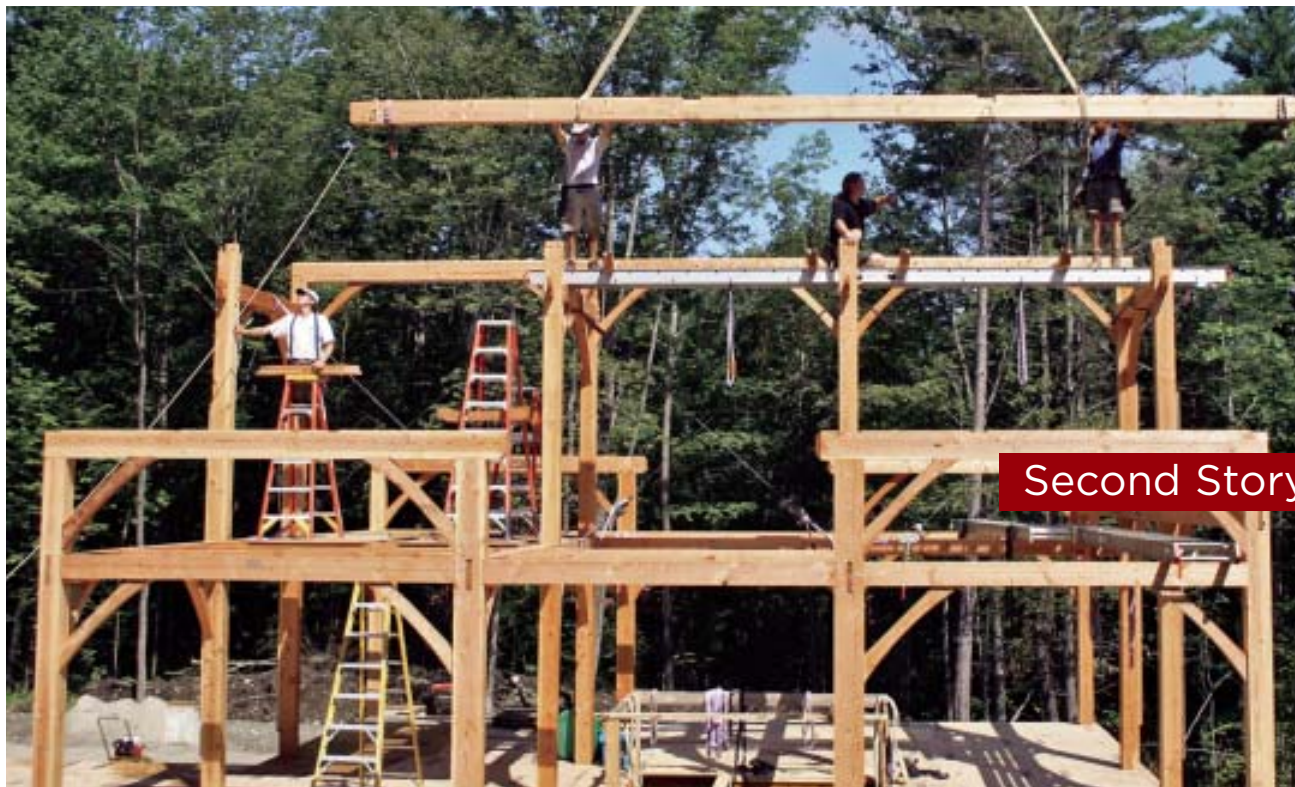
Figure 6. Assembly continues with the second-story posts and connecting plates (above), which are mortised to receive the rafters (far left). Braces are nailed along the outside of the perimeter posts, where the nail holes will not be visible (left).
