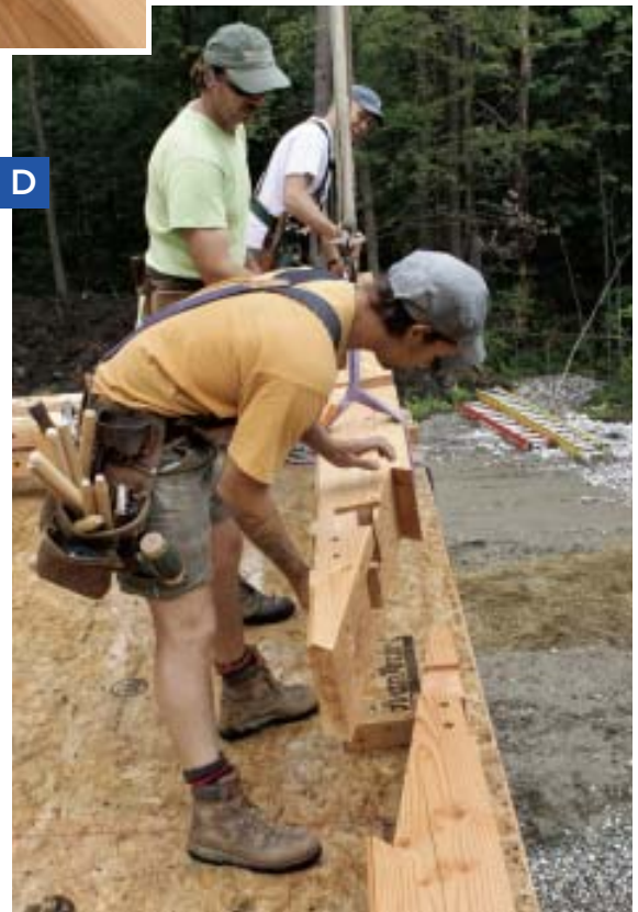
Figure 1. Housed mortises — like the one in the post cut to receive the knee brace (A) — help prevent members from twisting as they dry. Rafters have an interlocking joint at the top plate (B) and a pegged mortise-and-tenon joint at the peak (C). Long members, like plates that run the length of a wall, are made with scarf joints (D).
