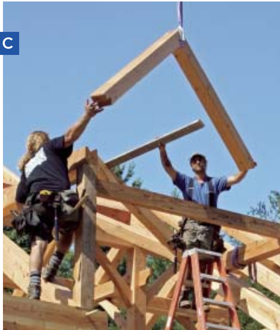
Figure 7. With small cleats tacked on top to prevent the straps from sliding, the rafters are lifted into place one at a time (A). After opposing rafters are pegged at the top, they are nailed to midspan purlins with long ring-shank nails (B). A gable dormer completes the frame (C, D).
