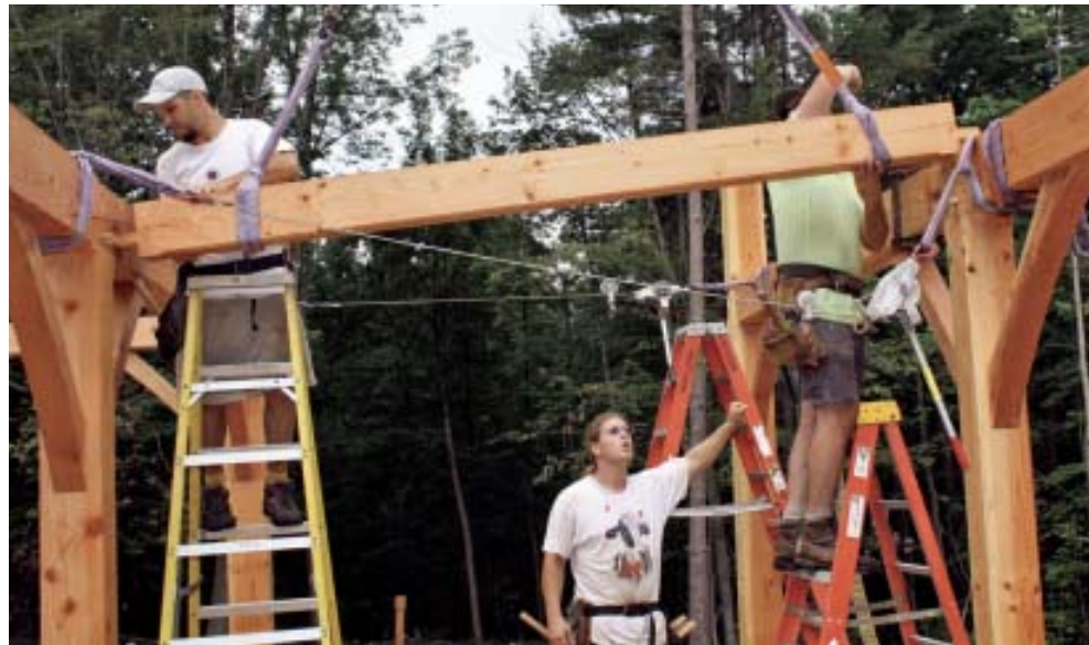
Figure 5. After a pair of bents has been raised and braced (above left), the crew uses come-alongs and the crane to cautiously spread the bents, coax the tenoned girts into their mortises, then pull the bents back together (above right and bottom).
