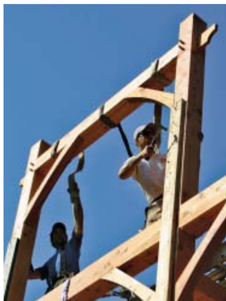
Figure 6. Assembly continues with the second-story posts and connecting plates (above), which are mortised to receive the rafters (far left). Braces are nailed along the outside of the perimeter posts, where the nail holes will not be visible (left).
