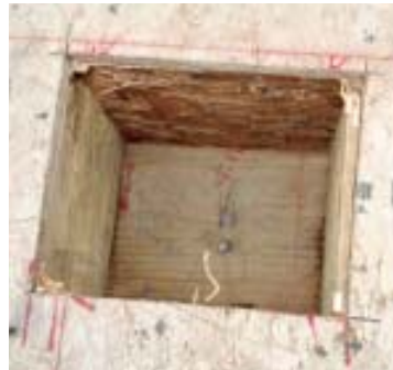
Figure 4. Assembling a frame starts with the bent farthest from the crane (top and far left). Carefully sized pockets in the subfloor (left) will receive the posts — a detail the author likes because it provides good bearing directly onto the sill and also helps prevent the posts from twisting.
