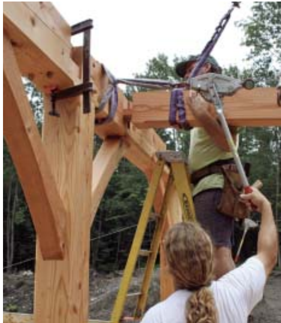
Figure 5. After a pair of bents has been raised and braced (above left), the crew uses come-alongs and the crane to cautiously spread the bents, coax the tenoned girts into their mortises, then pull the bents back together (above right and bottom).
