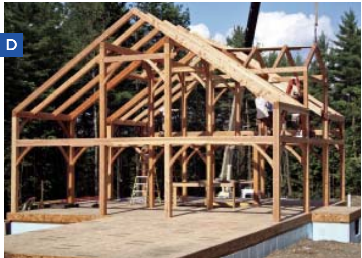
Figure 7. With small cleats tacked on top to prevent the straps from sliding, the rafters are lifted into place one at a time (A). After opposing rafters are pegged at the top, they are nailed to midspan purlins with long ring-shank nails (B). A gable dormer completes the frame (C, D).
