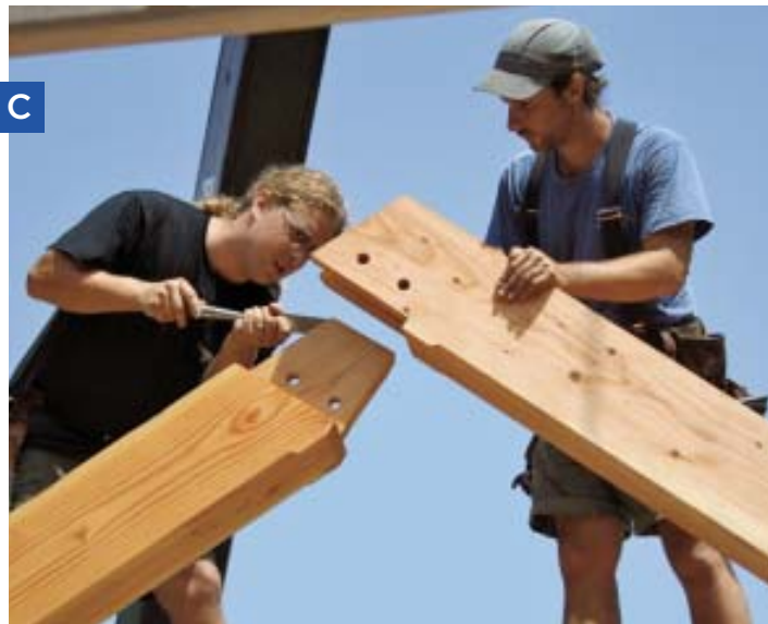
Figure 1. Housed mortises — like the one in the post cut to receive the knee brace (A) — help prevent members from twisting as they dry. Rafters have an interlocking joint at the top plate (B) and a pegged mortise-and-tenon joint at the peak (C). Long members, like plates that run the length of a wall, are made with scarf joints (D).
