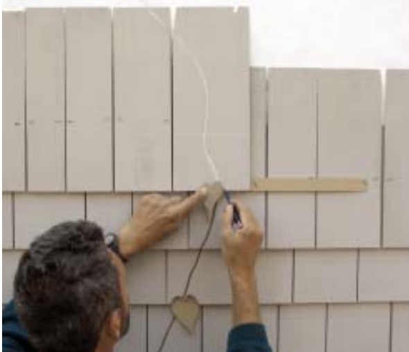
Figure 6. To complete the design, the author traces the leaf pattern onto an overlaying shingle and sketches in the route of the vine (above), then cuts out the top of the leaf and the vine slot (above right) before installing this shingle and the remaining field shingles (right).
