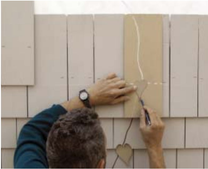
Figure 5. The author traces a leaf pattern onto a full-sized under-course shingle (above), then cuts out the exposed portion of the leaf with a jigsaw (above right). After fastening the leaf shingle in place, he fastens sideways shingle ramps on either side (right).
