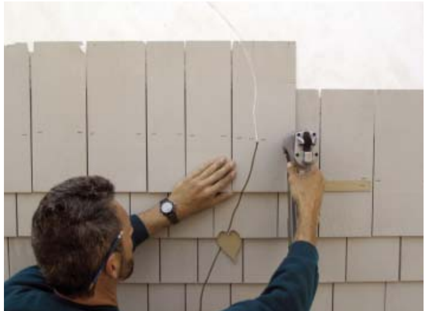
Figure 4. After marking the route for the vine (above), the author uses a jigsaw to cut the vine slot to a point just beyond the exposure line (above right). Extra fasteners at the vine slot help prevent the shingle from splitting (right).
