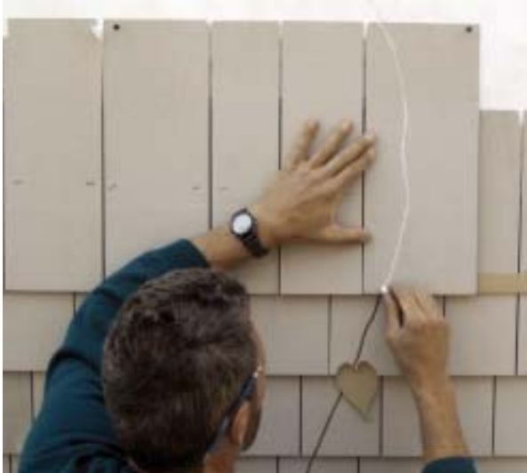
Figure 4. After marking the route for the vine (above), the author uses a jigsaw to cut the vine slot to a point just beyond the exposure line (above right). Extra fasteners at the vine slot help prevent the shingle from splitting (right).
