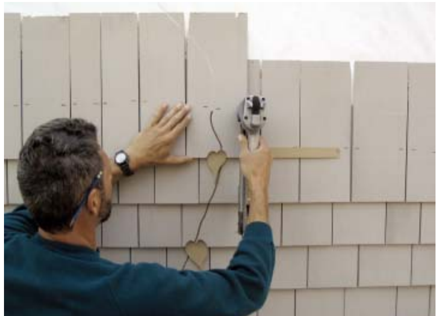
Figure 6. To complete the design, the author traces the leaf pattern onto an overlaying shingle and sketches in the route of the vine (above), then cuts out the top of the leaf and the vine slot (above right) before installing this shingle and the remaining field shingles (right).
