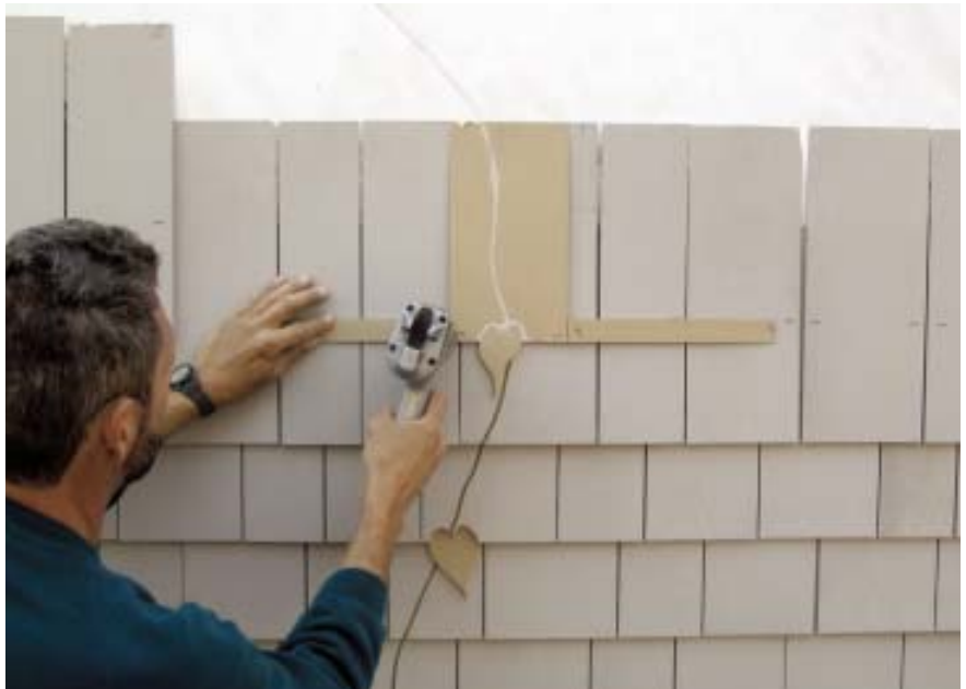
Figure 5. The author traces a leaf pattern onto a full-sized under-course shingle (above), then cuts out the exposed portion of the leaf with a jigsaw (above right). After fastening the leaf shingle in place, he fastens sideways shingle ramps on either side (right).
