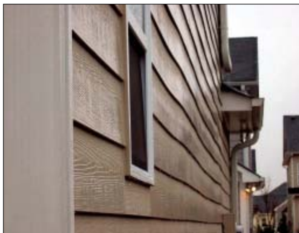
FIGURE 3. All wall and roof panels should be gapped to accommodate expansion of the panels. If installed too tightly, the panels can buckle the siding — a condition called “oil canning.”
