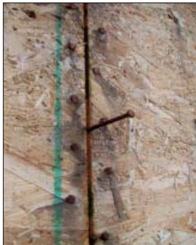
FIGURE 3. All wall and roof panels should be gapped to accommodate expansion of the panels. If installed too tightly, the panels can buckle the siding — a condition called “oil canning.”
