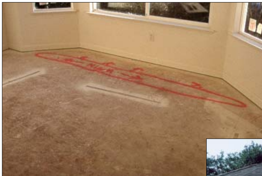
FIGURE 2. Panel swell is most sensitive along the edges where it is critical for flooring and roof sheathing to match up and not show through the finish flooring or roofing materials. At left, the edges of an OSB subfloor swelled significantly from rainwater blowing through window openings during construction. Below, the swelled edges of OSB sheathing show prominently through the shingles.
