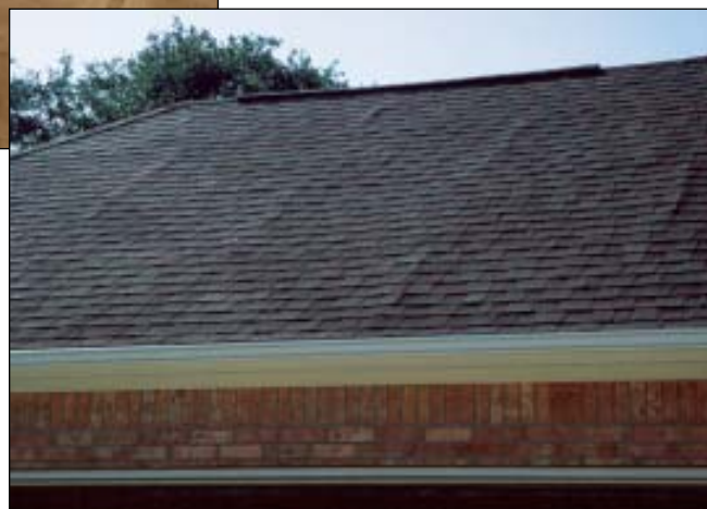
FIGURE 2. Panel swell is most sensitive along the edges where it is critical for flooring and roof sheathing to match up and not show through the finish flooring or roofing materials. At left, the edges of an OSB subfloor swelled significantly from rainwater blowing through window openings during construction. Below, the swelled edges of OSB sheathing show prominently through the shingles.
