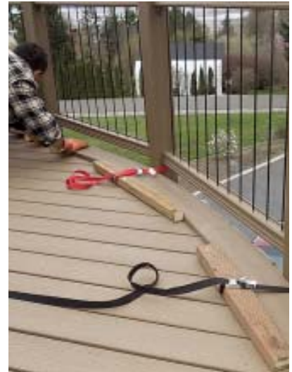
Figure 2. Pushed tight to the inside of the posts and secured with binder straps, the bent board is left to cool. Working to the inside of the posts bends the board to a slightly tighter radius, allowing for some “spring back” at installation.
