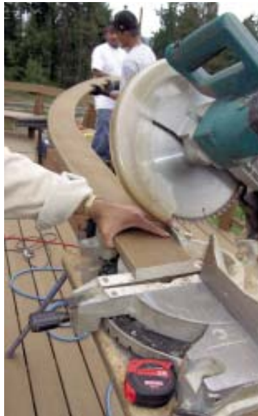
Figure 3. After its length is marked in place, the bent board is bevel-cut to be joined to another (left). The crew uses screws to attach the curved cap rail (right).
