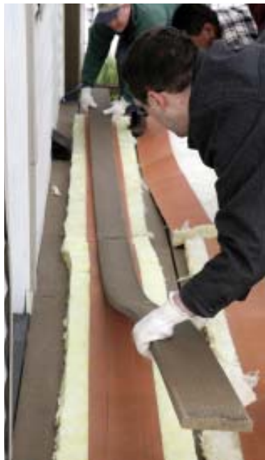
Figure 1. In about 40 minutes, heat pads raise the temperature of the composite board, making it bendable. Insulation above and below keeps in the warmth.
