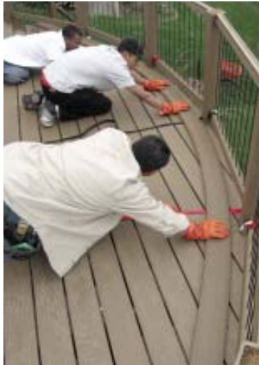
Figure 2. Pushed tight to the inside of the posts and secured with binder straps, the bent board is left to cool. Working to the inside of the posts bends the board to a slightly tighter radius, allowing for some “spring back” at installation.
