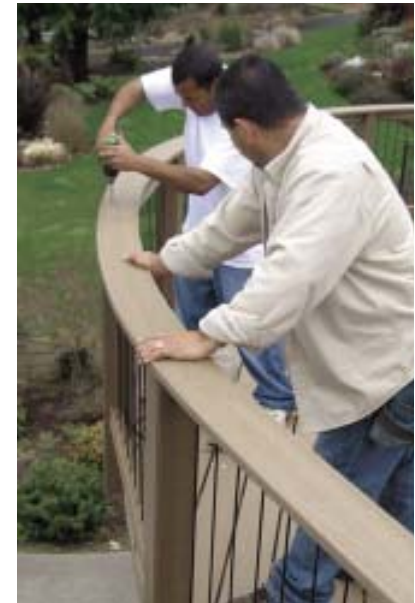
Figure 3. After its length is marked in place, the bent board is bevel-cut to be joined to another (left). The crew uses screws to attach the curved cap rail (right).
