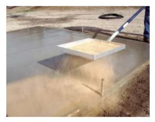
Powder Placer. Spreading the powdered dye and hardener used with concrete can create quite a mess — on your hands, your clothes, even your customer's landscaping. That's why contractor Brian Bettencourt invented the *Color Spreader*. The 18<sup>1</sup>/4-inch aluminum-framed, steel-meshed sifter lays down a 14-inch path of dye with every pass, and does so with greater consistency than hand-spreading, Bettencourt says. It attaches to standard screw-in or plug-in poles and sells for \$125.
