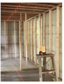
The PLS90E projects a pair of beams that fan out to form vertical planes of laser light exactly 90 degrees apart (left). Since the beams are plumb, the lines up the walls are plumb and the lines on the ceiling are directly over the lines on the floor (right).
