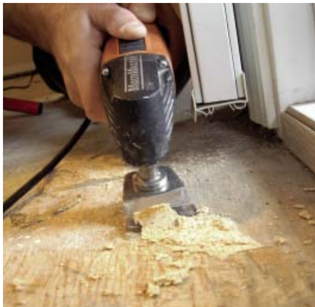
A scraper removes the stubborn remnants of particleboard underlayment. The MultiMaster's scraping blades can remove caulk, paint, vinyl flooring, and adhesives.
