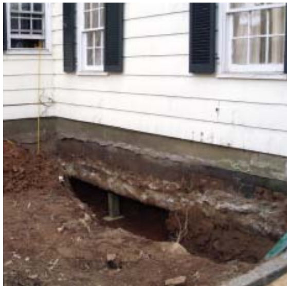
Figure 3. After digging a trench alongside the existing front-wall footing with an excavator, the author's crew used hand tools and a rotary hammer fitted with a chisel to remove the compacted soil under the footing (left). To prevent damage to the foundation, half the wall at a time was excavated and temporarily shored up (above).
