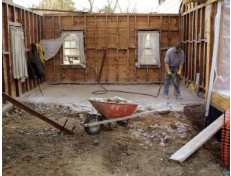
Figure 2. Before framing could begin, most of the existing garage had to be demolished, except for the sidewall — which was needed to retain the structure's 5-foot zoning variance — and the front wall, which needed to be reinforced with a deeper footing.
