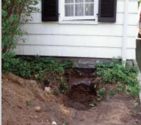
Figure 1. A test pit revealed that this shallow foundation footing, though adequate for a garage, could not support the loads created by the addition of second-floor living space without reinforcement.
