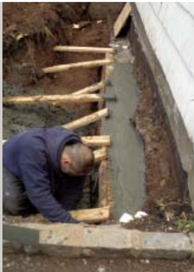
Figure 5. After stripping the form from the first half of the front-wall underpinning, the author's crew finished excavating underneath the remaining wall (above). Form pins helped hold the bottom of the form in place (above right), while 2-by-braces secured the top plate (right). The completed underpinning (far right).
