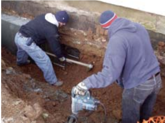
Figure 5. After stripping the form from the first half of the front-wall underpinning, the author's crew finished excavating underneath the remaining wall (above). Form pins helped hold the bottom of the form in place (above right), while 2-by-braces secured the top plate (right). The completed underpinning (far right).
