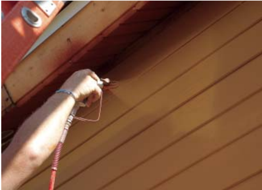
Figure 4. Maintain a vertical wet edge when you're spraying a second coat; it's a good way to keep track of what's already been sprayed.
