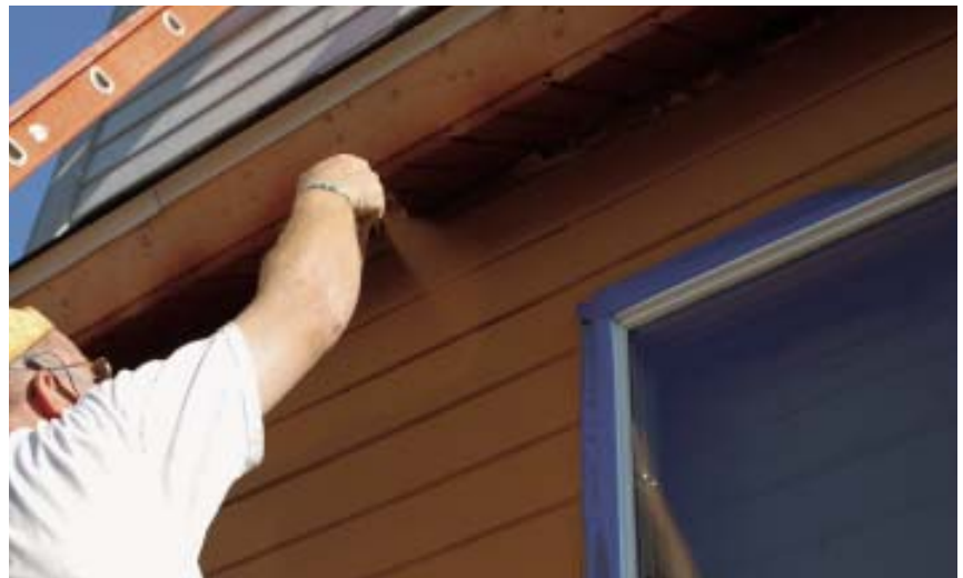
Figure 3. To apply an even coat, hold the gun parallel to the surface, whether moving horizontally (top left) or vertically (top right). When reaching high, make sure to maintain this position rather than angling the gun (above).
