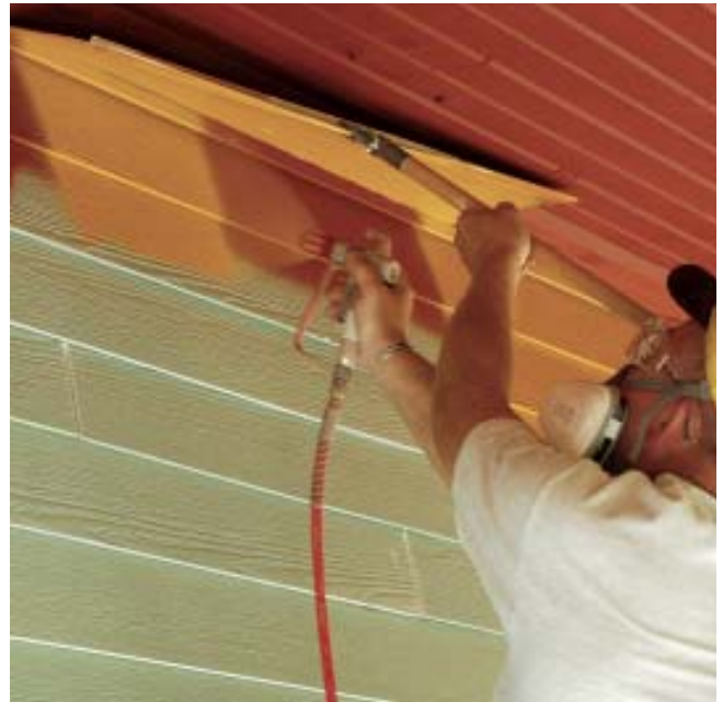
Figure 5. Taking the time to apply masking tape makes for fast cut-in (left). This hand-held masking tool (above) allows the author to cut in against a soffit of contrasting color with great accuracy.
