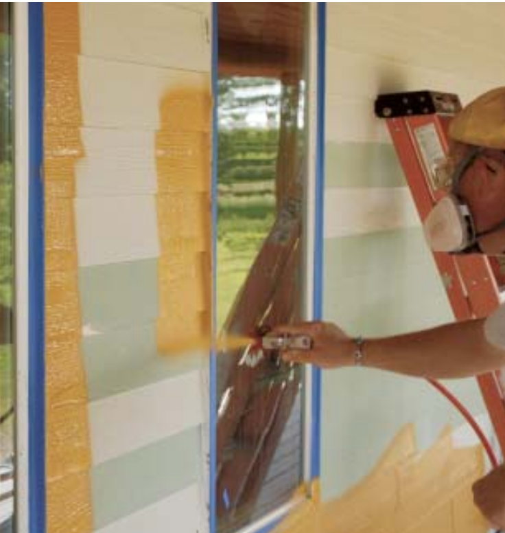
Figure 5. Taking the time to apply masking tape makes for fast cut-in (left). This hand-held masking tool (above) allows the author to cut in against a soffit of contrasting color with great accuracy.
