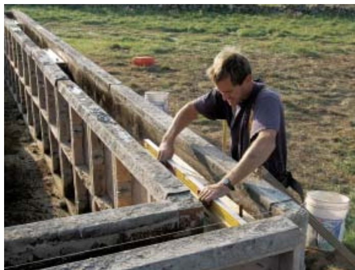
Figure 4. While the concrete is still plastic, the crew finds the lowest point on the foundation, then uses a sledge to tap all the plates to that elevation (far left). Here the author checks the short garage-wall plates for level (left).
