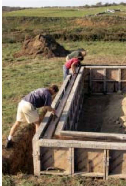
Figure 3. As the pour proceeds, the crew works quickly to position the plates (above left) and push the anchor bolts (above right and right).
