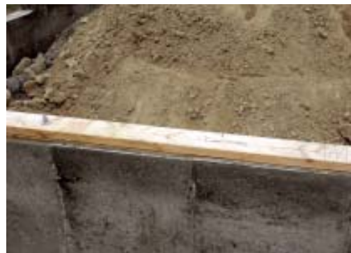
Figure 5. After the forms are stripped (above left), the author uses a claw hammer to remove the irregular ridge of concrete along the side of the sill (above). The finished result is accurately placed hold-down anchors and foundation bolts (left).
