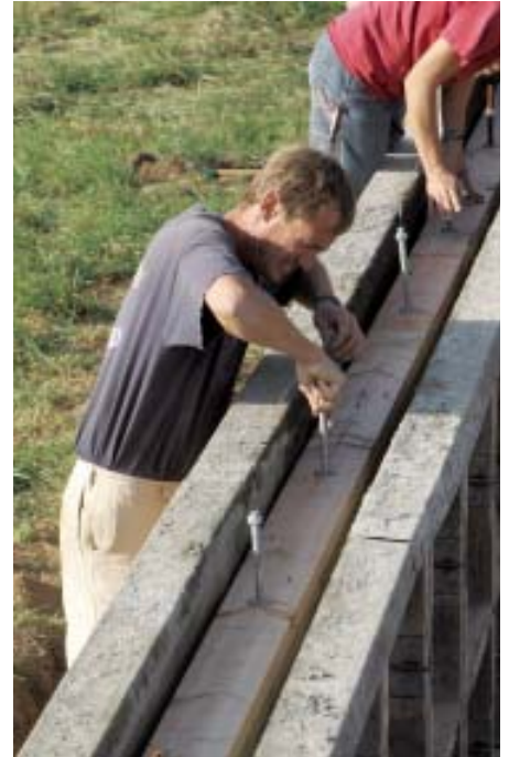
Figure 3. As the pour proceeds, the crew works quickly to position the plates (above left) and push the anchor bolts (above right and right).
