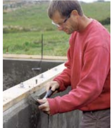
Figure 5. After the forms are stripped (above left), the author uses a claw hammer to remove the irregular ridge of concrete along the side of the sill (above). The finished result is accurately placed hold-down anchors and foundation bolts (left).
