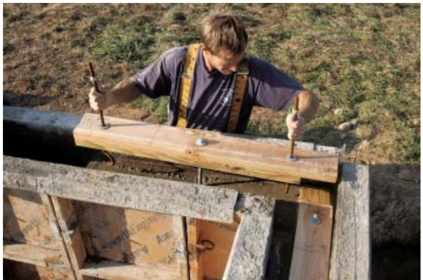
Figure 2. As soon as a section of wall is poured (top left), the author trowels the concrete to the correct level (top right). The plates — bolts and all — are then set into the wet concrete (above).
