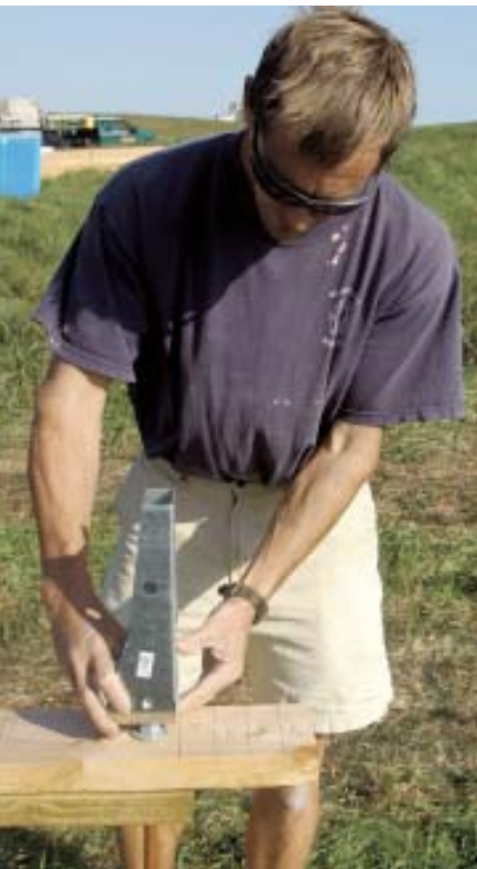
Figure 1. With the garage-wall bottom plate tacked to the mudsill, the author marks the stud layout, making adjustments as needed so that the anchor bolts don't interfere with the framing (top). He checks the placement of a hold-down bolt (above left) using the actual hardware, and labels each set of plates (above right) in preparation for concrete.
