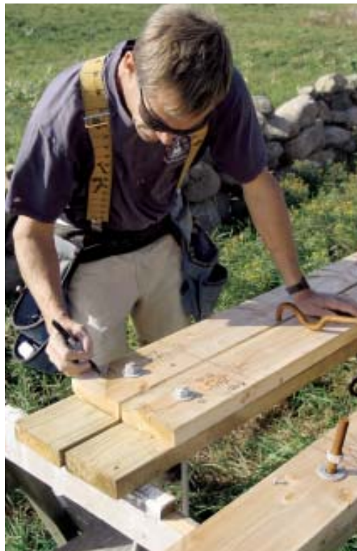
Figure 1. With the garage-wall bottom plate tacked to the mudsill, the author marks the stud layout, making adjustments as needed so that the anchor bolts don't interfere with the framing (top). He checks the placement of a hold-down bolt (above left) using the actual hardware, and labels each set of plates (above right) in preparation for concrete.
