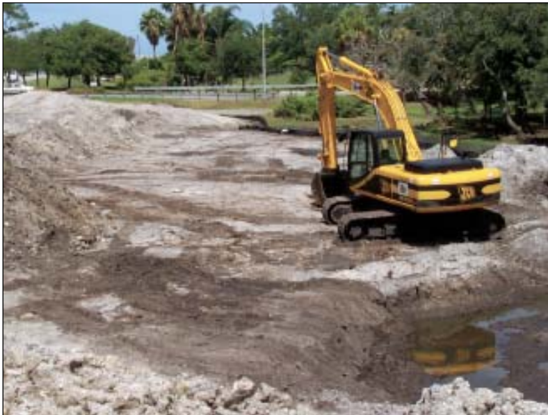
This wetlands in Sarasota County has been scraped to a level about 6 inches below the final grade. After this, a layer of organic matter will be laid in to provide a seed bed before the coffer dams are released at low tide to allow water to flow into the site.
