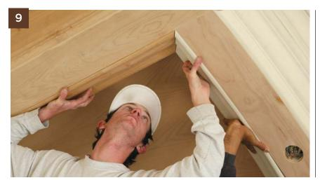
blocking to the ceiling with panel adhesive and nails. We waited a day for the adhesive to dry, then installed the sides of the beams, followed by the three-layered beam bottoms. We used <sup>1</sup>/<sub>4</sub>-inch MDF for the first two layers, and <sup>1</sup>/<sub>4</sub>-inch alder plywood for the exposed bottom layer.
