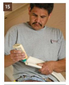
We used test pieces to check the fit of the miters (13), marked the length of each piece with the miter squeezed tightly in place (14), glued both sides of every miter (15), then sprung each piece into place, nailing off the miters and leaving a bow in the center, which we fastened last (16).
