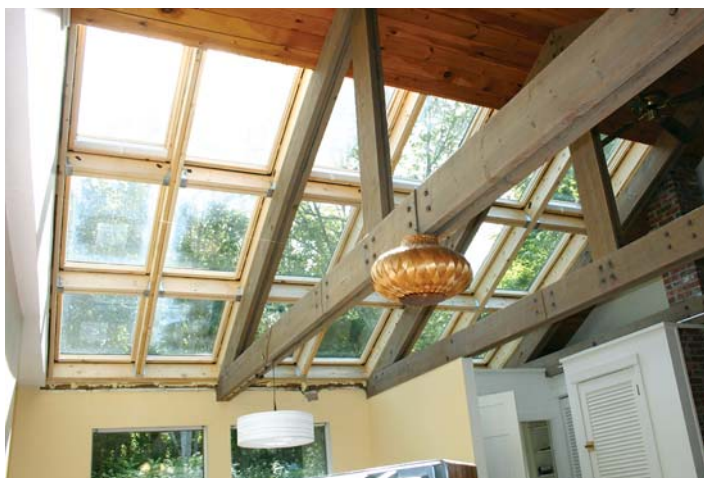
Figure 8. The 18 roof windows are a dramatic improvement — in both appearance and performance — over the original translucent plastic.
