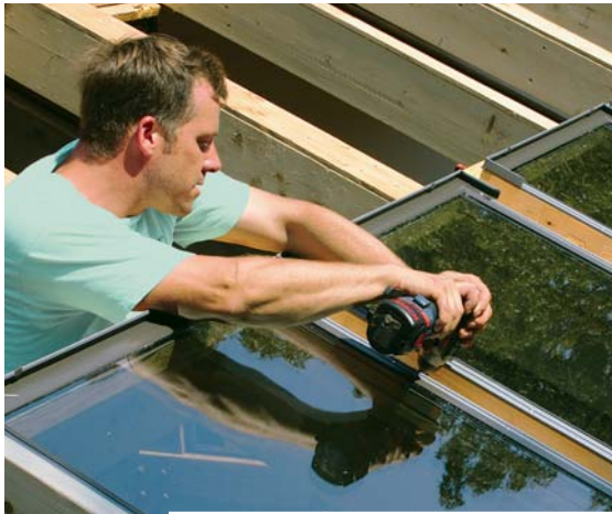
Figure 6. Access to the middle row of skylights was provided by staging inside the house (left) and, on the outside, a pair of planks spanning the installed bottom row (below). The 2x8 planks were attached to the roof framing with 12-inch-long timber screws. Intermediate support runners, secured to the planks with 6-inch bolts (bottom), gave additional support.
