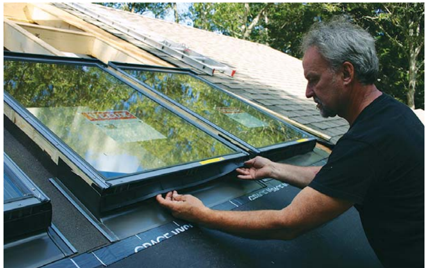
Figure 4. The head and apron flashings have an open hem (left) that engages an interlocking clip (below left), completing the water barrier. It's important to draw the rubber curb seal over the top of the apron flashing to prevent leaking (below right).
