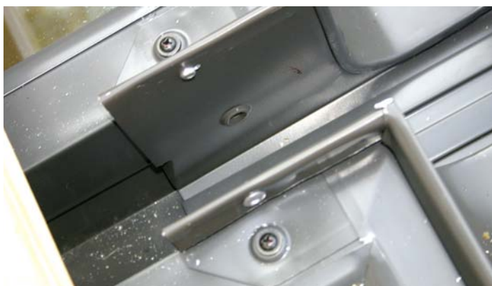
Figure 7. The combination head-sill flashings fit snugly in the 4-inch space between stacked units (left). Four small screws hold the finish cladding in place. A right-angle Phillips screwdriver (top) would make good standard equipment in the installation kit, since the author had to run out and locate one mid-job. Note the stainless steel rivets (above) — the author's solution for securing the head flashing because there wasn't enough room between units to insert a screw in the dimple along the side.
