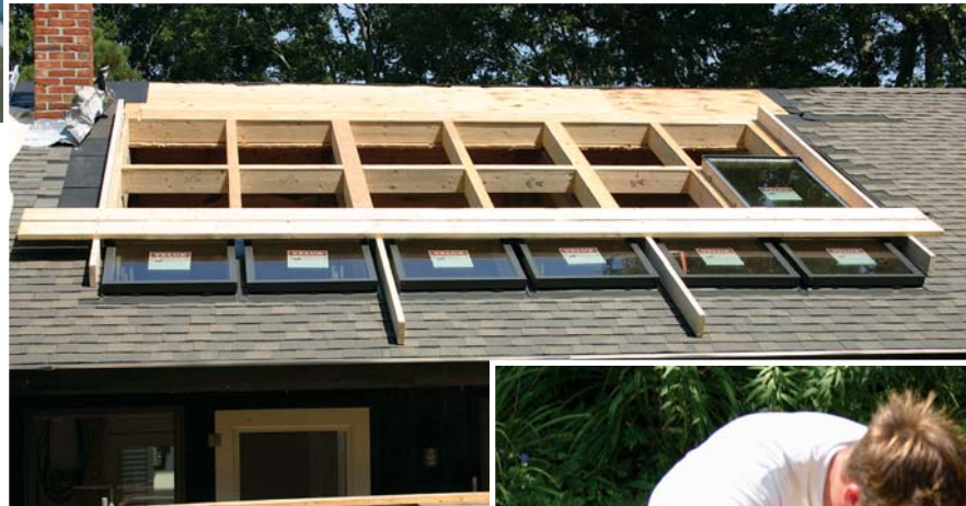
Figure 6. Access to the middle row of skylights was provided by staging inside the house (left) and, on the outside, a pair of planks spanning the installed bottom row (below). The 2x8 planks were attached to the roof framing with 12-inch-long timber screws. Intermediate support runners, secured to the planks with 6-inch bolts (bottom), gave additional support.
