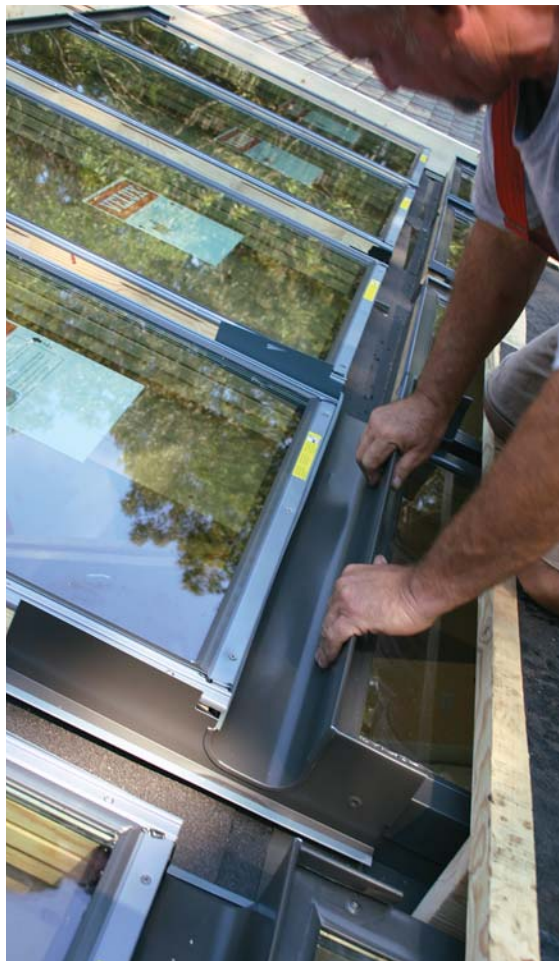
Figure 7. The combination head-sill flashings fit snugly in the 4-inch space between stacked units (left). Four small screws hold the finish cladding in place. A right-angle Phillips screwdriver (top) would make good standard equipment in the installation kit, since the author had to run out and locate one mid-job. Note the stainless steel rivets (above) — the author's solution for securing the head flashing because there wasn't enough room between units to insert a screw in the dimple along the side.
