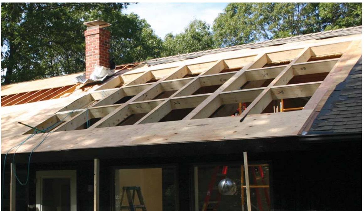
Figure 1. The original rough opening (left) was almost perfectly square, a lucky start on a project that demanded accurate framing (below).
