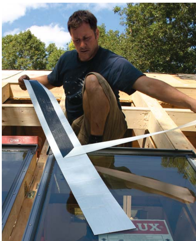
Figure 3. U-shaped and L-shaped pieces of self-sticking roofing membrane seal the transition between roof and frame (top). The author cut strips from a 3-foot-wide roll of ArmourGard Ice & Water Protector, then scored the release sheet so it could be peeled away a section at a time — first the middle (above), then the sides (right).
