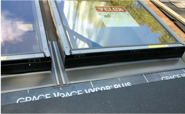
Figure 4. The head and apron flashings have an open hem (left) that engages an interlocking clip (below left), completing the water barrier. It's important to draw the rubber curb seal over the top of the apron flashing to prevent leaking (below right).
