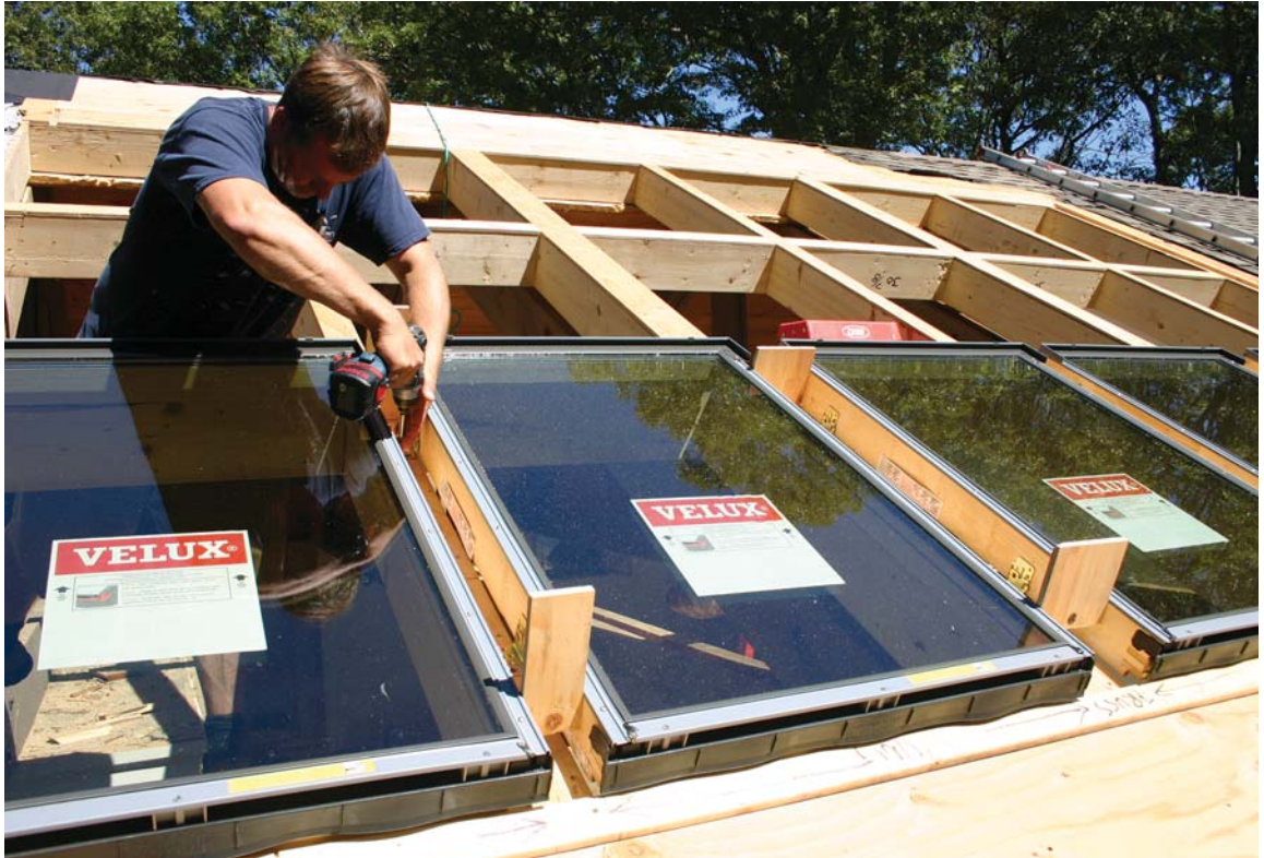
Figure 2. The author laid out the units and the flashing spaces between them on a 1x3 story stick that he nailed to the roof to guide framing. Here, the stick is screwed to a chalk line below the completed rough opening to support and position the bottom row of windows. Plywood gauges ensure accurate spacing between the window frames and prevent dimensional creep.
