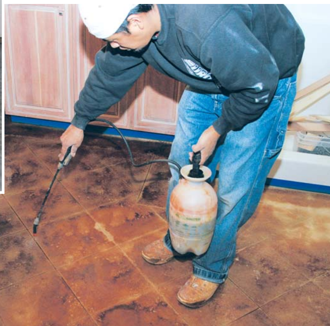
Figure 5. A crew member applies acid stain with a chemically resistant hand sprayer (left). After the acid reaction is complete, it's possible to touch up areas that haven't darkened enough (below).
