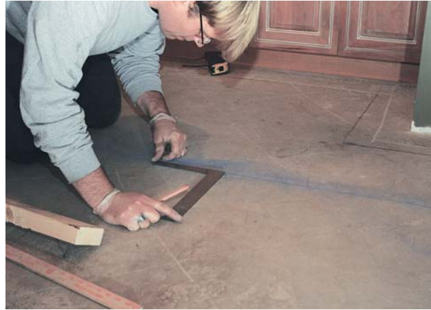
Figure 2. The scored tile grid is drawn freehand, then snapped out in chalk. Before cutting, the author fine-tunes the pattern in pencil using squares and straightedges. Here, he avoids having to cut in tight corners by including a 6-inch border around the bathroom cabinets.
