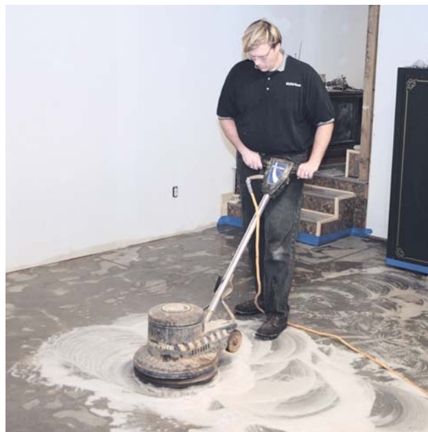
Figure 4. The author spreads stripper with a mop (above left), then buffs the wet floor with a medium-grit pad and a screen to lift the concrete sealer (above). Residual stripper is picked up with a wet vac (far left). A floor may need several applications before all the sealer lifts; trouble spots (left) require experimenting with a variety of chemicals.
