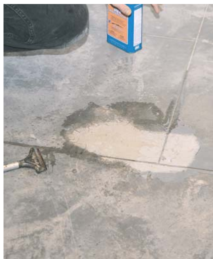
Figure 4. The author spreads stripper with a mop (above left), then buffs the wet floor with a medium-grit pad and a screen to lift the concrete sealer (above). Residual stripper is picked up with a wet vac (far left). A floor may need several applications before all the sealer lifts; trouble spots (left) require experimenting with a variety of chemicals.
