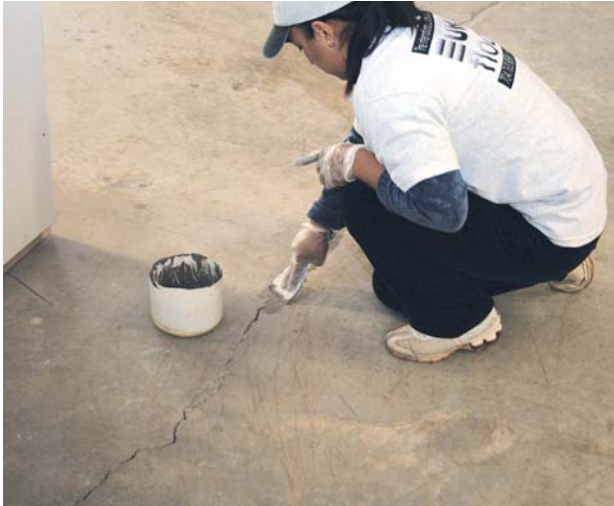
Figure 1. The first step in the staining process is to fill any pronounced cracks in the slab with a Portland cement-based patching compound. After staining, the cracks create a marbled effect.
