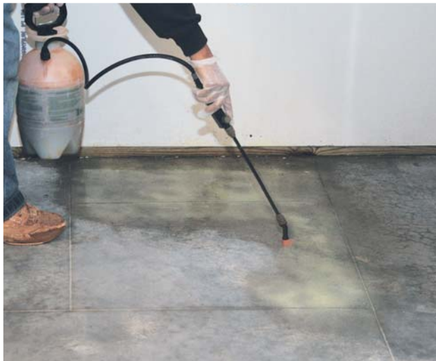
Figure 5. A crew member applies acid stain with a chemically resistant hand sprayer (left). After the acid reaction is complete, it's possible to touch up areas that haven't darkened enough (below).
