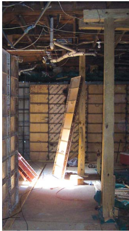
Figure 4. Pressure-treated 2x4s shot into the footing restrained the bottom of the one-sided wall forms (left); diagonal braces secured to temporary posts and the floor framing above held the top and middle (right).
