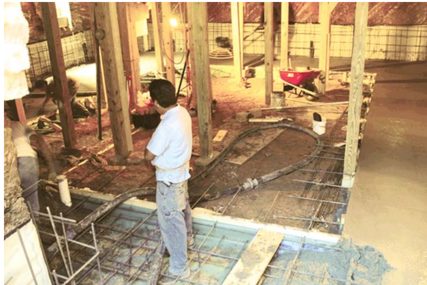
Figure 2. Shown here (top) is the first of two layers of rebar designed to tie the 6-foot-wide footing to the new concrete walls, creating an 8-foot retaining wall inside the basement. The concrete was pumped in (above), then power-troweled for a smooth finish (left).
