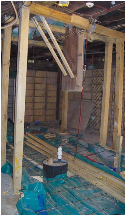
Figure 5. The new bathroom required a sewage ejector pump (left), which is located in the middle of one of the footings designed for the basement's bearing walls (above).
