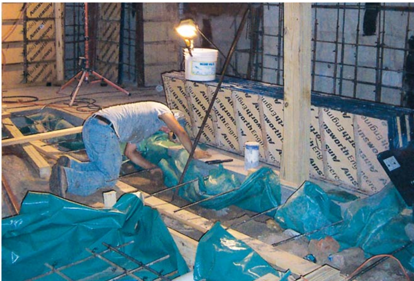
Figure 3. Before the walls could be poured, the waterproofing subcontractor installed MiraDrain and MiraClay membranes all the way to the top of the excavation (top left), then covered the exposed dirt at the top with a poly vapor barrier (top right). He also spread poly over the dirt floor in preparation for placing the slab (above).
