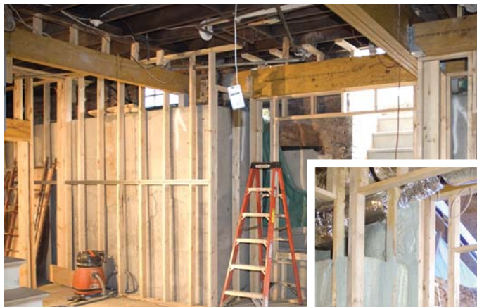
Figure 6. LVL beams now support the first floor, with room above for mechanicals (left). New stud walls around the perimeter were insulated with high-density polyurethane sprayed directly against the new concrete and existing brick (below left). The new space includes two egress windows (below right) and a large exercise and media room (bottom).
