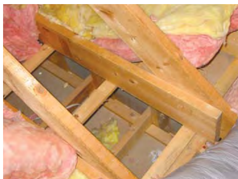
Figure 6. Moving attic insulation uncovers a common cause of leaks: wire holes through partition-wall top plates (above). The double line of soot stains indicates upward air leaks between the drywall and a partition plate (top right). Fiberglass stuffed into a plumbing wall (center right) was no match for the air rising from below; note the spray foam at left in the photo — the solution. A double layer of fiberglass did not prevent air movement through an interior soffit into the attic (bottom right).
