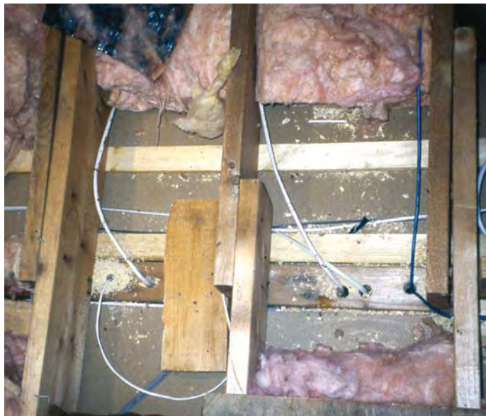
Figure 6. Moving attic insulation uncovers a common cause of leaks: wire holes through partition-wall top plates (above). The double line of soot stains indicates upward air leaks between the drywall and a partition plate (top right). Fiberglass stuffed into a plumbing wall (center right) was no match for the air rising from below; note the spray foam at left in the photo — the solution. A double layer of fiberglass did not prevent air movement through an interior soffit into the attic (bottom right).
