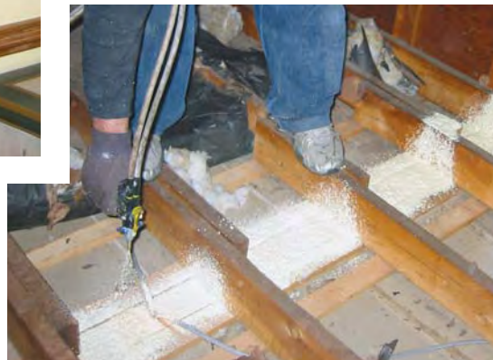
Figure 5. The infrared scan revealed an unexpected cold area in this interior partition wall, which was traced to air leaking into the attic along the top plate, shown here being sealed (right).
