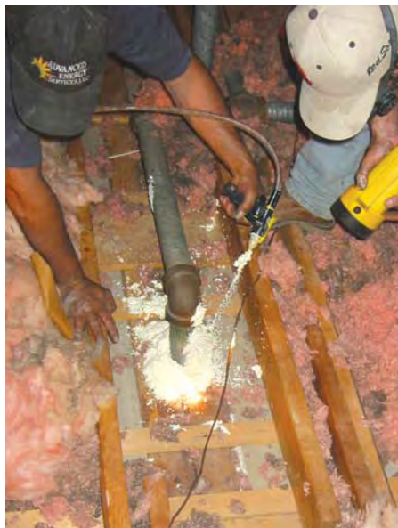
Figure 7. Because it sticks even to dirty surfaces, two-part urethane foam works well for sealing around attic penetrations (left). A worker seals beneath an attic ledger (above), after first chinking the gap underneath with fiberglass.
