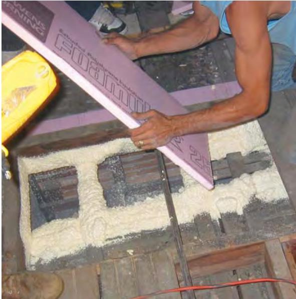
Figure 8. Rigid foam board is ideal for sealing large openings like this oversized framing chase. After cutting the board to fit, the worker beds it in wet spray foam (left), then seals the edges (above).
