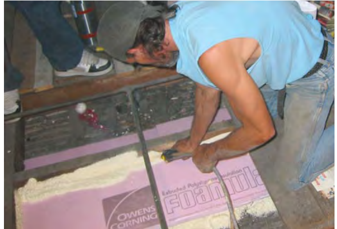
Figure 8. Rigid foam board is ideal for sealing large openings like this oversized framing chase. After cutting the board to fit, the worker beds it in wet spray foam (left), then seals the edges (above).
