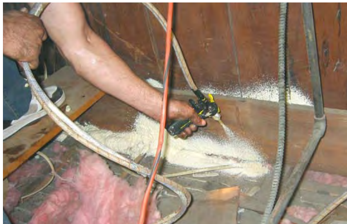
Figure 7. Because it sticks even to dirty surfaces, two-part urethane foam works well for sealing around attic penetrations (left). A worker seals beneath an attic ledger (above), after first chinking the gap underneath with fiberglass.
