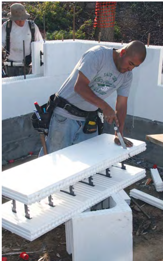
Figure 1. To minimize cutting, the crew works from the corners toward the middle of the wall and fills in the last piece. Here a carpenter trims (left) and installs (above) the last block in a course.
