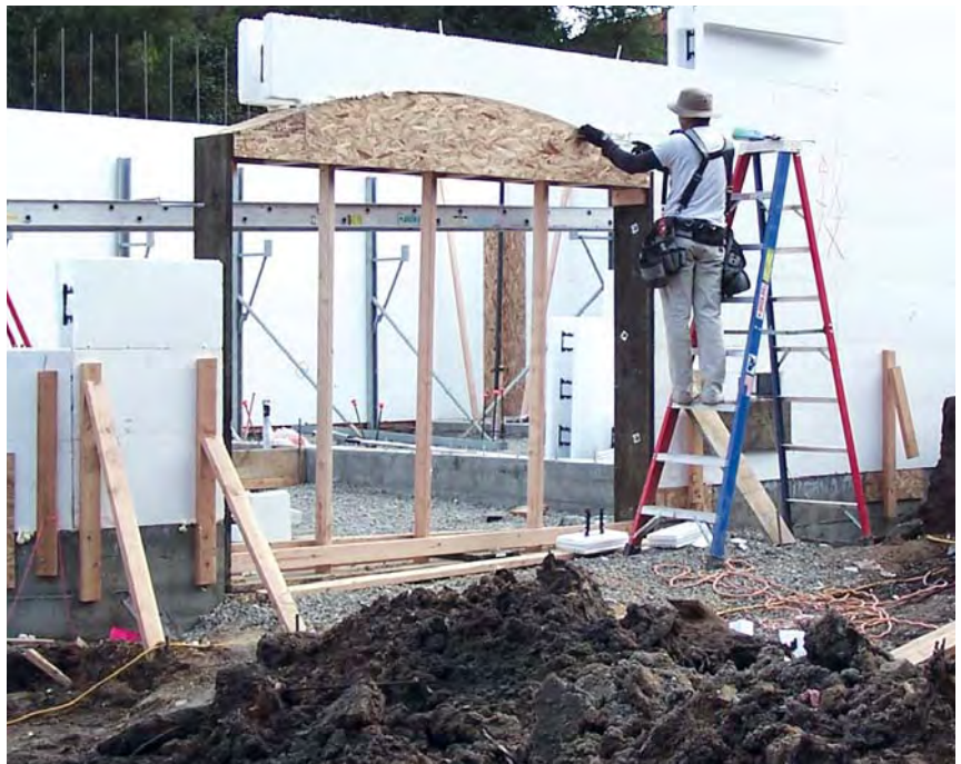
Figure 5. Carpenters plumb and brace the buck for an arch-top window (top). The buck for the garage opening is supported on a temporary stud wall; the pressure-treated side jambs will remain in place for fastening the overhead door tracks (above).
