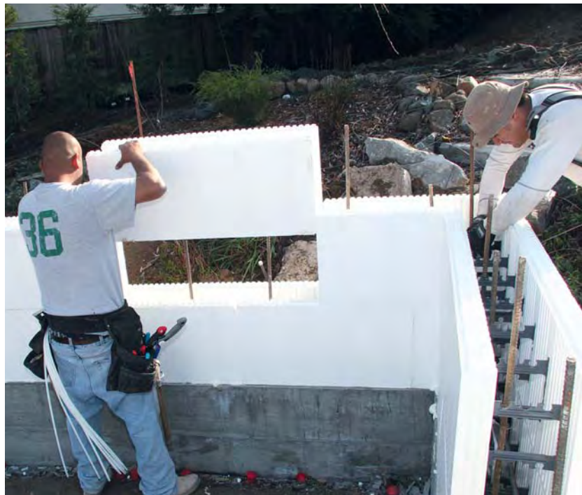
Figure 1. To minimize cutting, the crew works from the corners toward the middle of the wall and fills in the last piece. Here a carpenter trims (left) and installs (above) the last block in a course.
