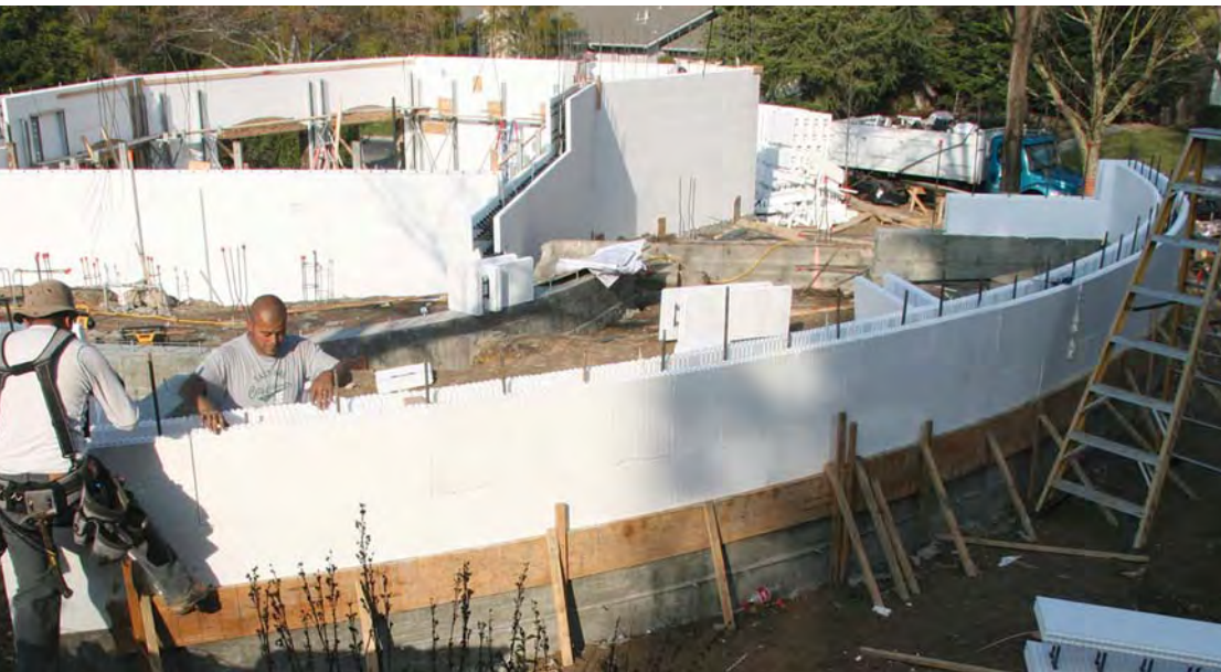
Figure 3. The crew creates the curve by cutting the inside faces of the block slightly shorter than the outside faces and flexing the pieces into an arc. Kerfed 2x10 braces hold the bottom course in line with the grade beam.
