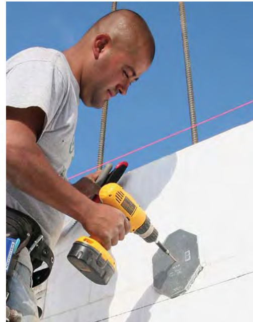
Figure 4. The upper floor hangs from ledgers attached with Simpson hardware designed for ICFs. The legs of the metal plate — punched so that they will key into the concrete — are inserted into slots in the foam (above left), then the plate is fastened with a screw so it can't fall out during the pour (above). After the concrete cures, the ledger is positioned against the wall and fastened to the plate with structural screws driven through a special hanger (left).
