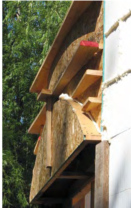
Figure 7. The arched bucks in curved walls were made extra wide to accommodate the radius.
