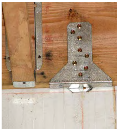
Figure 4. The upper floor hangs from ledgers attached with Simpson hardware designed for ICFs. The legs of the metal plate — punched so that they will key into the concrete — are inserted into slots in the foam (above left), then the plate is fastened with a screw so it can't fall out during the pour (above). After the concrete cures, the ledger is positioned against the wall and fastened to the plate with structural screws driven through a special hanger (left).
