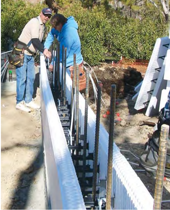
Figure 2. The author prefers to fasten the first two courses together (above), using zip ties (above right). He then straightens and levels the two courses as a unit, which he glues to the footing with spray foam (right).
