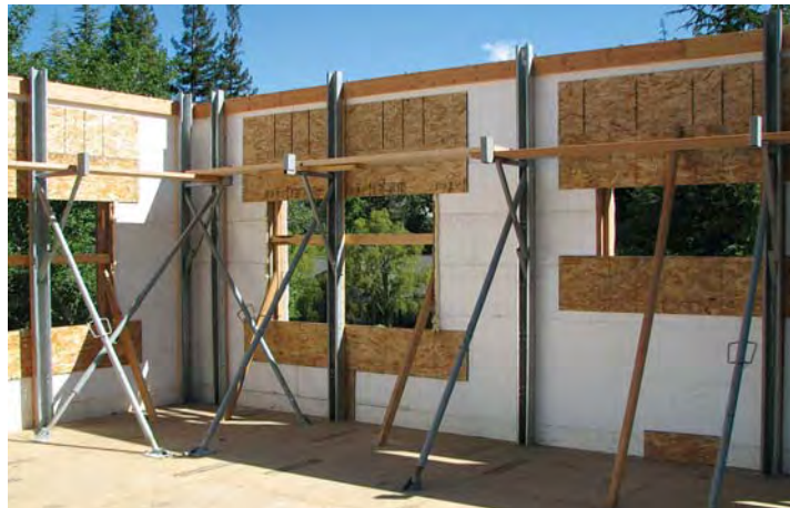
Figure 8. In preparation for concrete, the window bucks were reinforced with additional pieces of OSB and the wall thoroughly braced.
