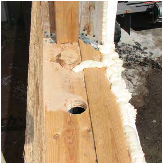
Figure 6. To make it easy to remove, this window buck was assembled from the inside with framing angles and screws. Note the sloped sill; the inspection holes allow carpenters to verify that concrete has filled the blocks below.
