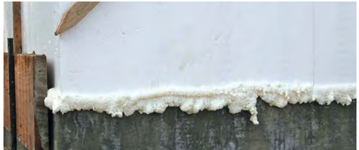
Figure 2. The author prefers to fasten the first two courses together (above), using zip ties (above right). He then straightens and levels the two courses as a unit, which he glues to the footing with spray foam (right).
