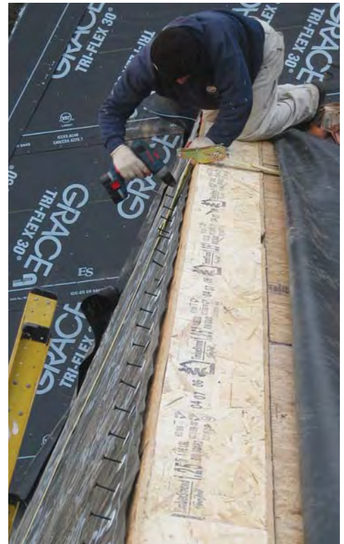
Figure 4. With the main roof sections fastened together, the adjoining hips are installed (above left). To save time, the author's crew preinstalls the connecting screws on the ground before lifting the panels into position (above), and preassembles small hip sections before placement (left).
