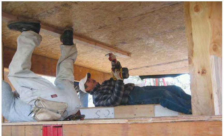
Figure 2. Roof sections are assembled and prepped on the ground; sealing the panel joints with asphalt cement helps prevent the OSB skins from absorbing moisture and swelling, while extra strips of underlayment laid over the patch keeps the tar under control (left). Placing the panels on 30-inch-tall LVL sawhorses allows crew members to work underneath (below). After assembly, each section is rigged with lifting straps and hoisted into place with an all-terrain forklift (bottom).
