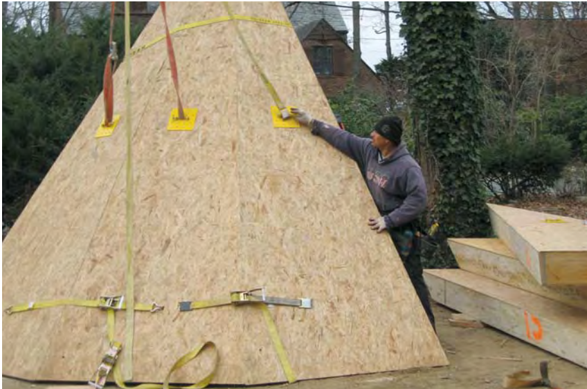
Figure 6. Small and large turrets are assembled on the ground out of pre-cut SIPs (right) and then hoisted into place with the forklift (below). The radius-roofed dormers — which were preassembled at the factory — are lifted straight from the delivery truck to the roof (bottom).
