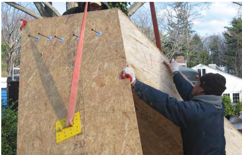
Figure 4. With the main roof sections fastened together, the adjoining hips are installed (above left). To save time, the author's crew preinstalls the connecting screws on the ground before lifting the panels into position (above), and preassembles small hip sections before placement (left).
