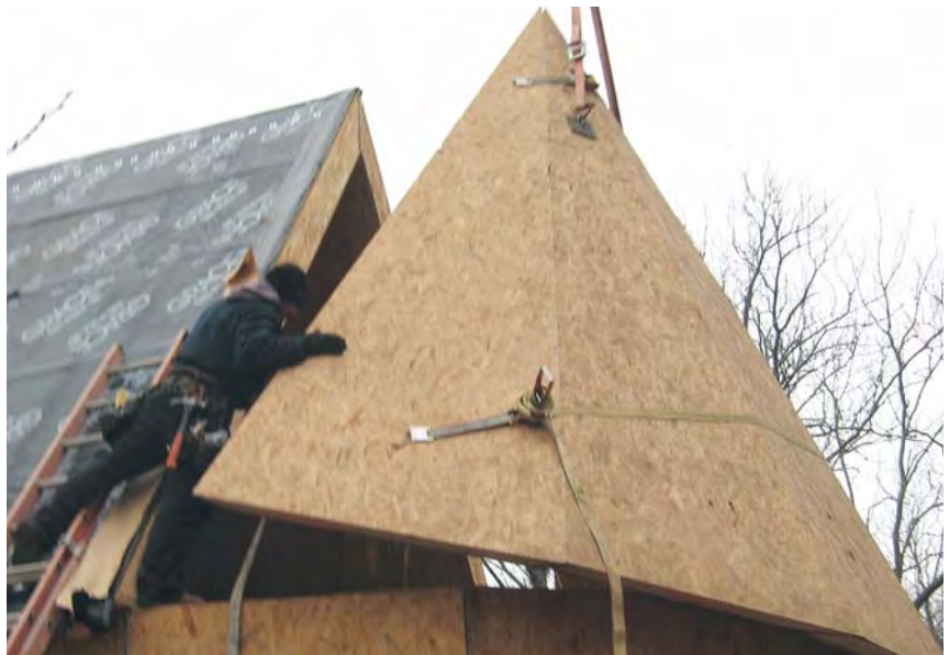
Figure 6. Small and large turrets are assembled on the ground out of pre-cut SIPs (right) and then hoisted into place with the forklift (below). The radius-roofed dormers — which were preassembled at the factory — are lifted straight from the delivery truck to the roof (bottom).
