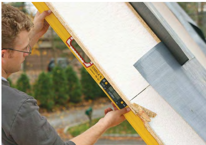
Figure 3. To set the first roof section, the author projects the centerline of the ridge connection (marked on the deck) with a vertical laser line, then props the section into position with the forklift (top). After the roof pitch is verified with a digital level (above), the section is temporarily braced until the opposing roof section can be rigged and set into place.
