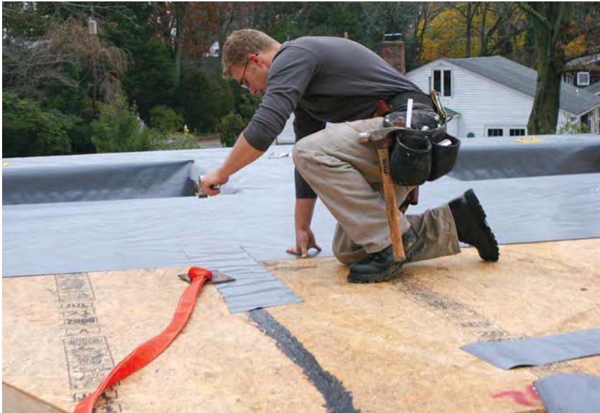
Figure 2. Roof sections are assembled and prepped on the ground; sealing the panel joints with asphalt cement helps prevent the OSB skins from absorbing moisture and swelling, while extra strips of underlayment laid over the patch keeps the tar under control (left). Placing the panels on 30-inch-tall LVL sawhorses allows crew members to work underneath (below). After assembly, each section is rigged with lifting straps and hoisted into place with an all-terrain forklift (bottom).
