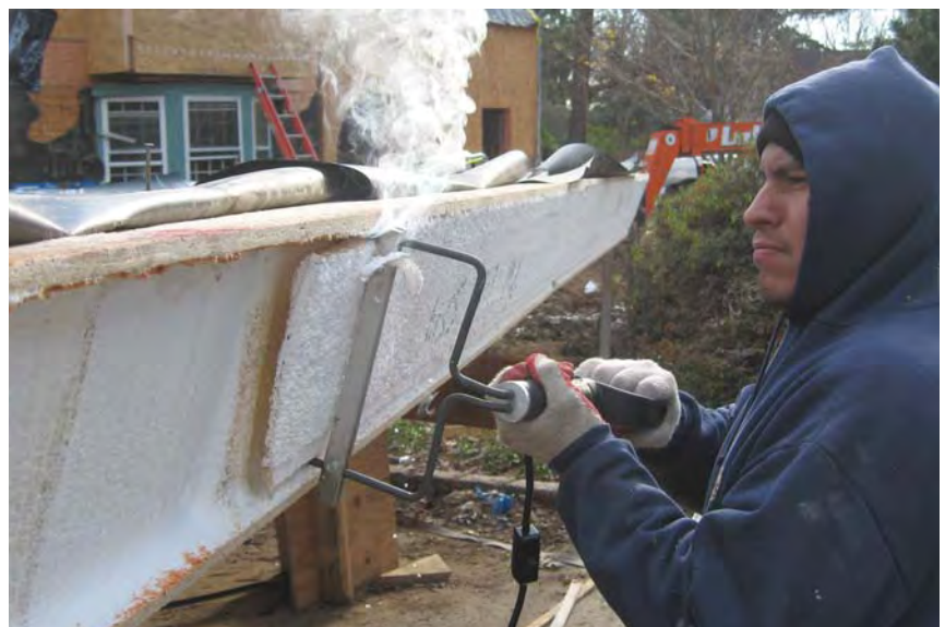
Figure 5. When a panel has been trimmed in the field, foam must be removed with a hot iron to make room for new blocking.
