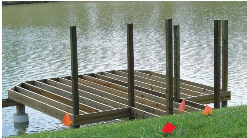
Figure 8. Once the outer footers and posts are complete, framing proceeds as it would with any freestanding deck.
