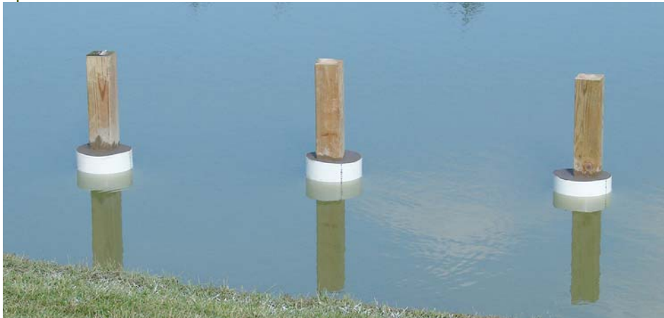
Figure 7. The outer posts are trimmed to the correct height after the concrete sets. White paint on the grass represents the maximum water level of the lake; the height of the framing should be several inches above that. The author uses a laser level to transfer this elevation from the shore to the posts.
