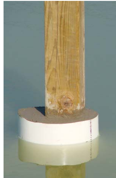
Figure 3. Large-diameter PVC pipe serves as a concrete form for the footers. The author extends it several inches above the average waterline.
