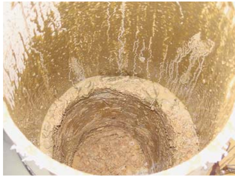
Figure 5. Once the PVC pipe is driven into the mud, it's emptied of water with a bucket. The footer is dug down into solid ground using a post-hole digger.
