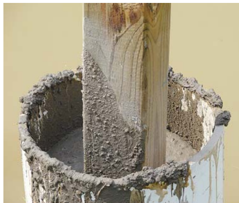
Figure 6. The 6x6 posts are set in the PVC forms and concrete is carried out from the shore in buckets and placed around the posts. The PVC will be trimmed to the level of the concrete with a cordless reciprocating saw after the concrete sets.
