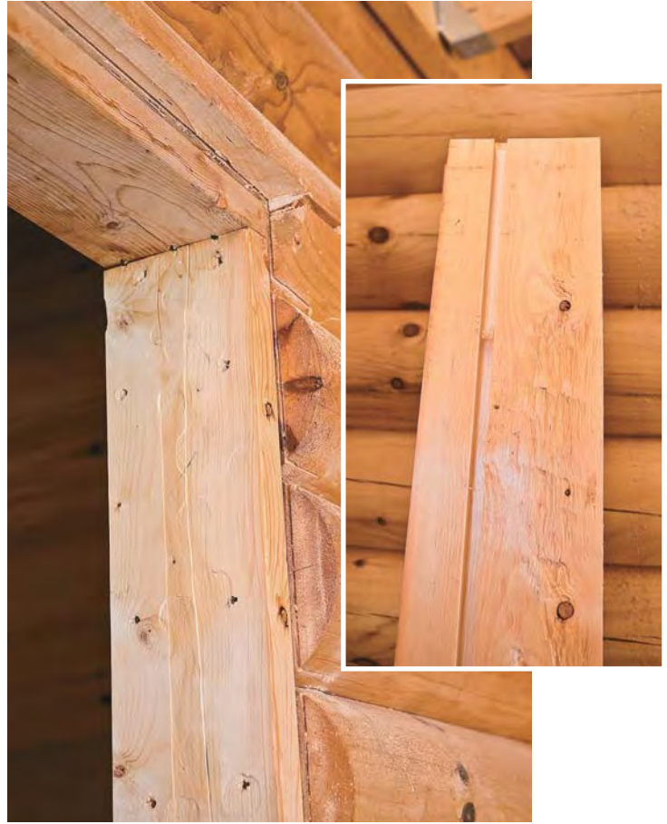
Figure 7. A carpenter taps in plywood splines (above left) that mate with dados in the backs of door and window bucks (above). The window fins are fastened to the bucks, then covered with trim (left).
