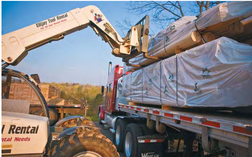
Figure 1. The author rents an all-terrain forklift on delivery days. The pallets are covered with plastic and arranged so the lower log courses are on top of the stack.
