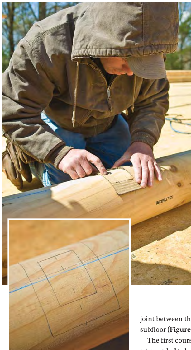
Figure 6. Using a cardboard template, a worker draws the outline of a work box (left), then uses a 1/2-inch drill with a Forstner bit to hog out the material (above). A small router finishes off the recess.
