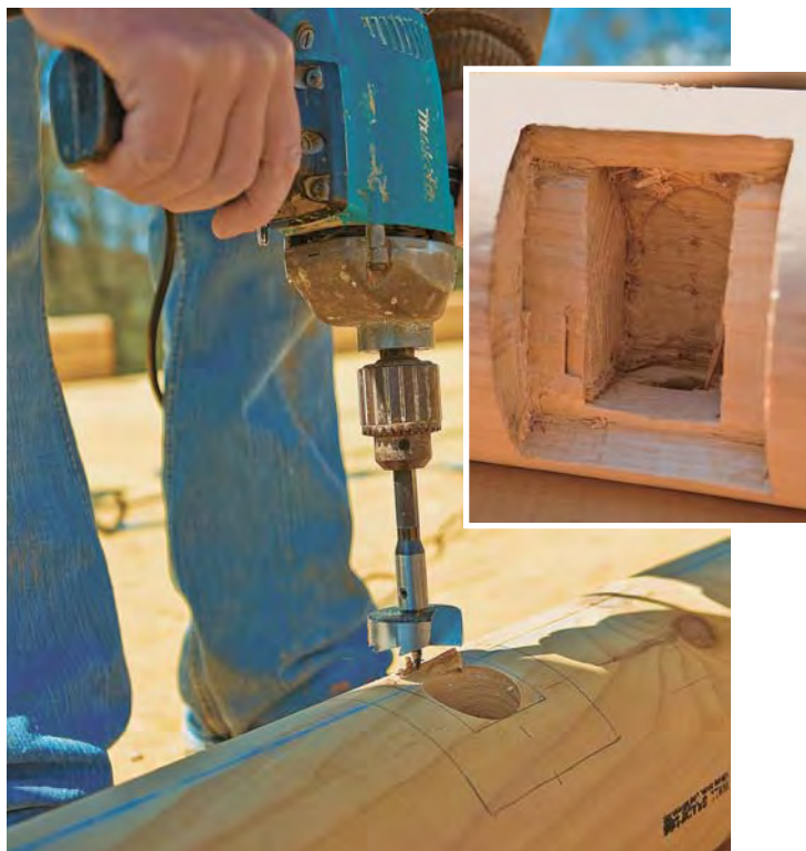
Figure 6. Using a cardboard template, a worker draws the outline of a work box (left), then uses a 1/2-inch drill with a Forstner bit to hog out the material (above). A small router finishes off the recess.
