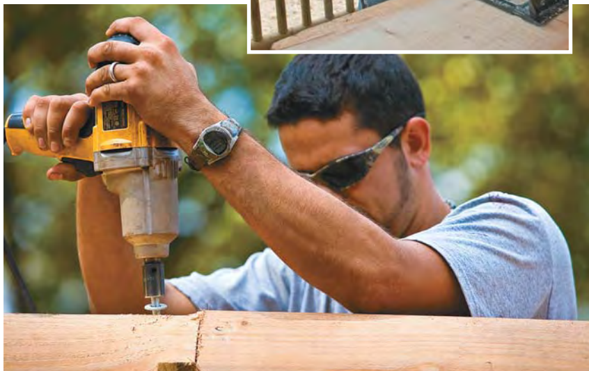
Figure 2. In addition to standard carpentry tools, building with logs requires a large circular saw for trimming ends and adding or expanding window and door openings. A 1/2-inch electric impact wrench drives the lag screws that connect the log courses.
