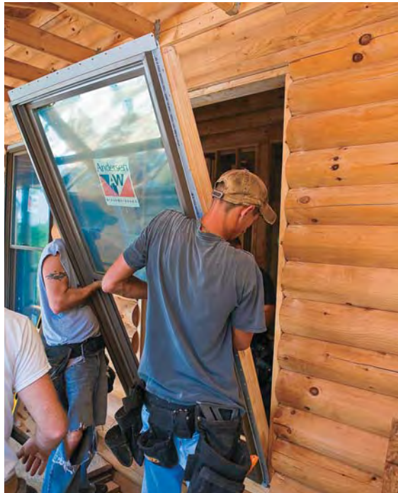
Figure 7. A carpenter taps in plywood splines (above left) that mate with dados in the backs of door and window bucks (above). The window fins are fastened to the bucks, then covered with trim (left).
