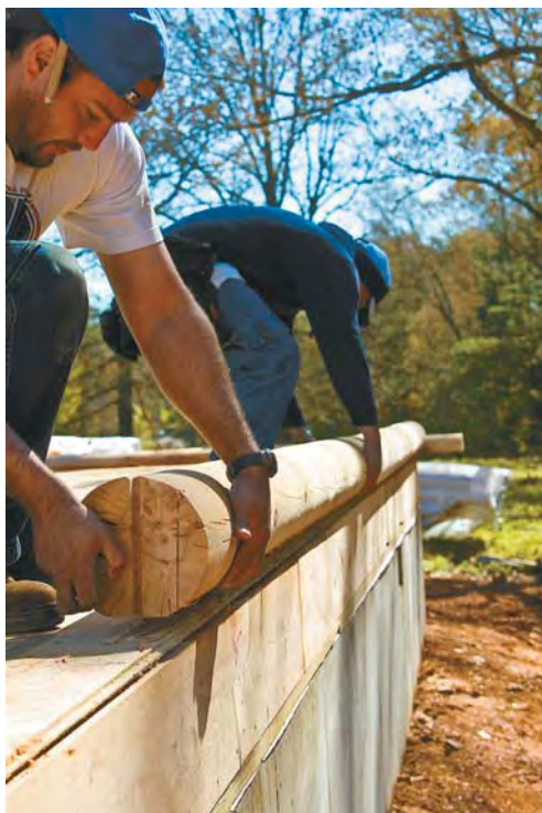
Figure 3. Set into urethane sealant, the first log course is carefully aligned to the layout lines with a framing or layout square. The ends of logs have dados that receive plywood splines for structural reinforcement and weatherproofing. While this wall starts with a full log, adjoining walls start with a half log so they can overlap at corners.
