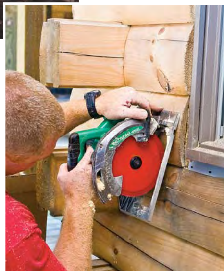
Figure 8. Doors and windows are cased with pine trim to match the logs. The preassembled picture-frame casing is scribed and let in over the window's nailing fin. A layer of peel-and-stick flashing over the fin seals the joint.
