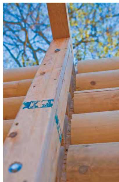
Figure 5. Where stick-framed interior walls meet the log walls, saw kerfs make it easy to install drywall or paneling that doesn't require fussy finishing or scribing. The kerfs are made on site with a circular saw and a chisel.
