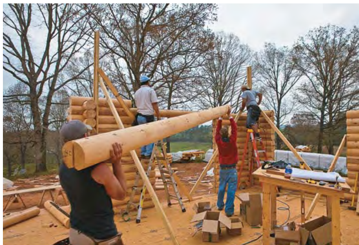
Figure 4. Dried to about 19 percent moisture content, kiln-dried logs are noticeably lighter than green logs. Most can be carried and lifted into place without struggle by a pair of workers. Logs are identified on their ends, and a framing plan provided by the manufacturer shows their location in the structure. T-shaped braces hold the walls plumb while they're assembled.
