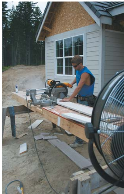
Figure 4. A sliding-compound miter saw equipped with a Hitachi fiber-cement blade cuts quickly but does a poor job of directing dust into the vacuum hose (left). A powerful fan (right) directs dust away from the operator toward an area where no one is working.
