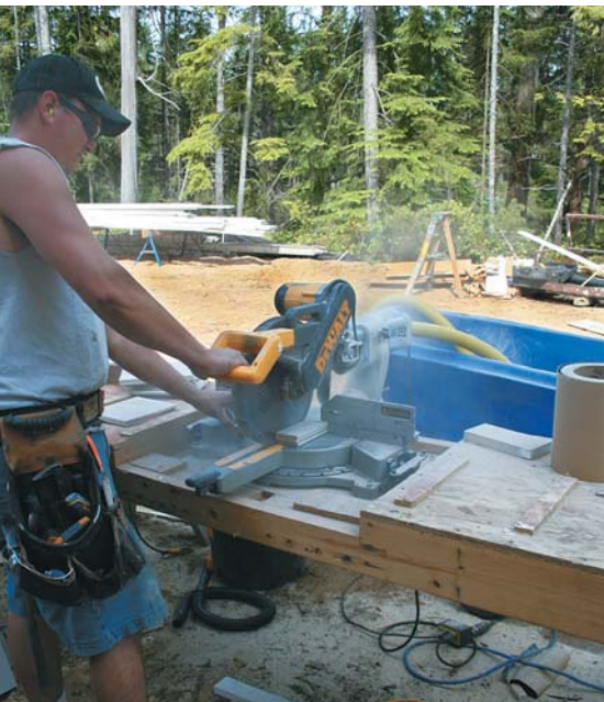
Figure 4. A sliding-compound miter saw equipped with a Hitachi fiber-cement blade cuts quickly but does a poor job of directing dust into the vacuum hose (left). A powerful fan (right) directs dust away from the operator toward an area where no one is working.
