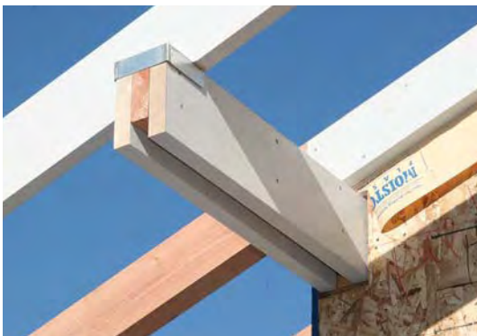
Figure 2. Triple 2-by members passing through the stick-framed gable walls form the 4-foot support purlins for the deep overhangs. An upside-down beam hanger secured to solid framing on the inside (above) helps resist rotation forces, and a cap flashing protects the exposed horizontal surface at the top end of each purlin.
