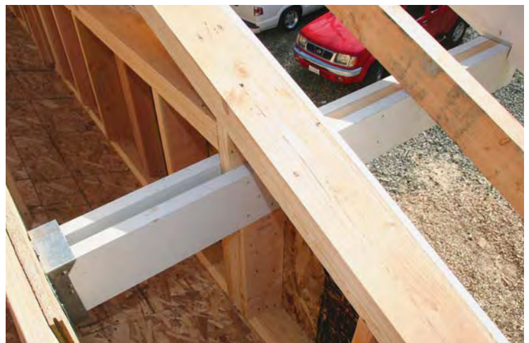
Figure 2. Triple 2-by members passing through the stick-framed gable walls form the 4-foot support purlins for the deep overhangs. An upside-down beam hanger secured to solid framing on the inside (above) helps resist rotation forces, and a cap flashing protects the exposed horizontal surface at the top end of each purlin.
