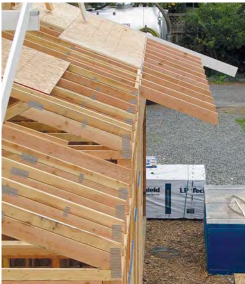
Figure 3. Three-by-six false rafter tails nailed to the top chords of the snub-end trusses penetrate the wall sheathing to create the appearance of an open-eaves stick-framed roof. They're positioned 1 inch below the top of the trusses so that the 2x6 roof planking to be installed over the eaves will be flush with the 1/2-inch OSB on the rest of the roof.
