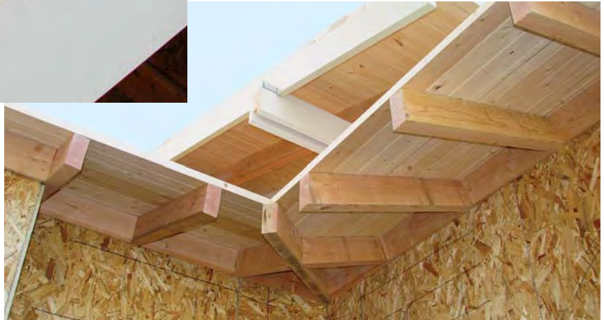
Figure 4. Two-by-six beveled-edge T&G pine completes the stick-framed look. At bottom, the completed house before painting.
