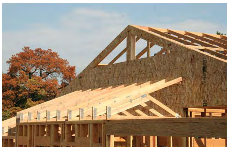
Figure 1. To make it easier to add the architect-designed 4-foot gable overhangs and 3-foot rafter tails along the eaves, the author stick-framed the gable walls and used snub-end trusses for the main roof.
