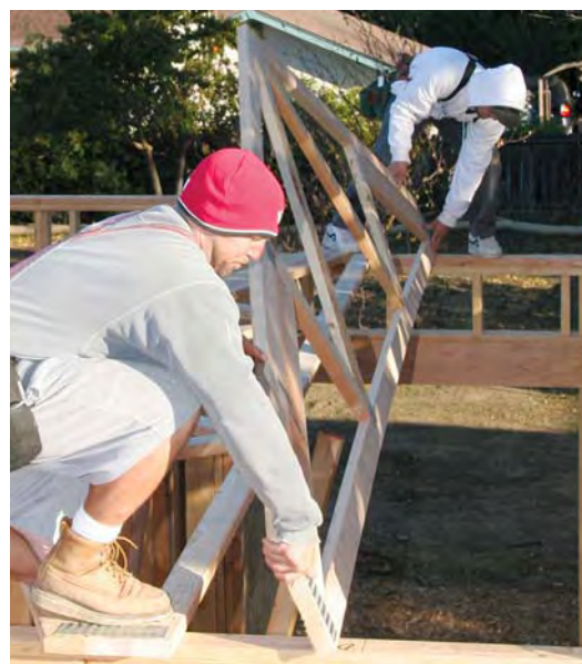
Figure 1. To make it easier to add the architect-designed 4-foot gable overhangs and 3-foot rafter tails along the eaves, the author stick-framed the gable walls and used snub-end trusses for the main roof.
