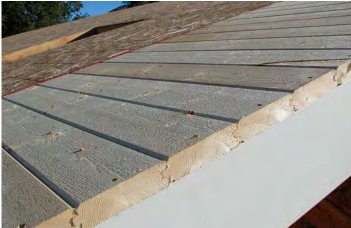
Figure 4. Two-by-six beveled-edge T&G pine completes the stick-framed look. At bottom, the completed house before painting.
