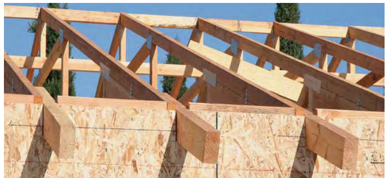
Figure 3. Three-by-six false rafter tails nailed to the top chords of the snub-end trusses penetrate the wall sheathing to create the appearance of an open-eaves stick-framed roof. They're positioned 1 inch below the top of the trusses so that the 2x6 roof planking to be installed over the eaves will be flush with the 1/2-inch OSB on the rest of the roof.
