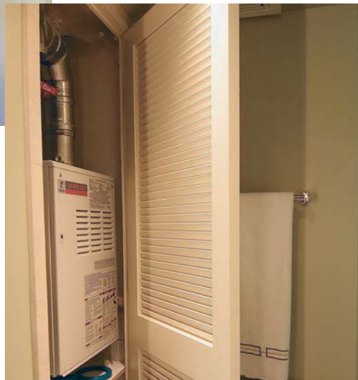
Figure 4. The original water heater was replaced with a tankless model, which sits in a shallow cabinet beside the wall-hung toilet. The cabinet door just clears the top of the fixture and is louvered to admit combustion air.
