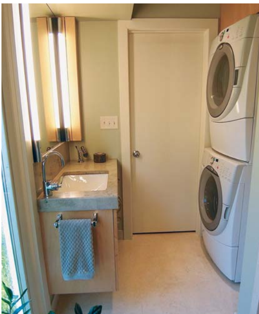
Figure 3. A washer and dryer stack in a niche at the end of the room. The wood panel above the appliances can be removed to access and clean the dryer vent.
