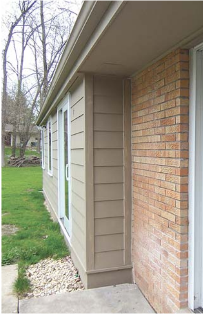
Figure 2. Valuable inches were gained by substituting fiber-cement siding for the original 5-inch brick veneer. The water table — which comes to within a couple of inches of grade — is made from cellular PVC, which won't rot or absorb water.
