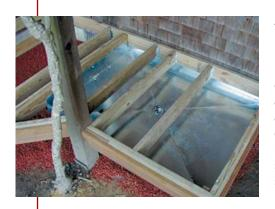
Appropriate drainage is a must. Local health codes may require the drains to lead into the sanitary sewers. Many areas, however, allow gray water to drain to a simple drywell. For belowdeck systems, the author has a local sheet-metal shop fabricate a galvanized-steel drain pan.
