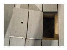
Access for cleaning debris, such as wind-blown leaves, is crucial. A simple hatch lifted by way of a thumbhole is all you need.
