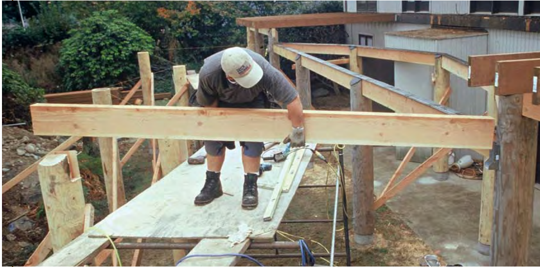
Figure 11. Before the beams are placed in their pockets, the wood is treated with a borate preservative. Note the torch-down roofing membrane applied to the beam and post tops in the background.
