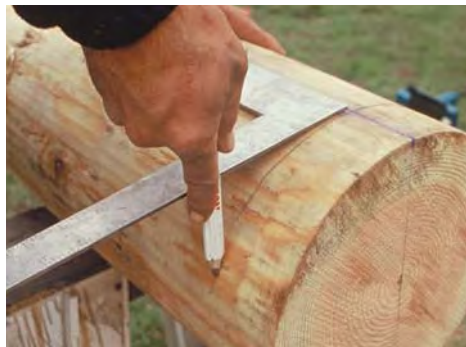
Figure 3. To mark the end of the log to be cut square to the centerline, a framing square is held to the layout line (left). It takes a little finesse to hold the pencil square to the square. After the cut, check for square (below), but remember to allow for any taper the log may have.
