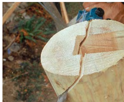
Figure 10. To shed water, the tops of the posts are beveled after the pockets for the beams are cut.
