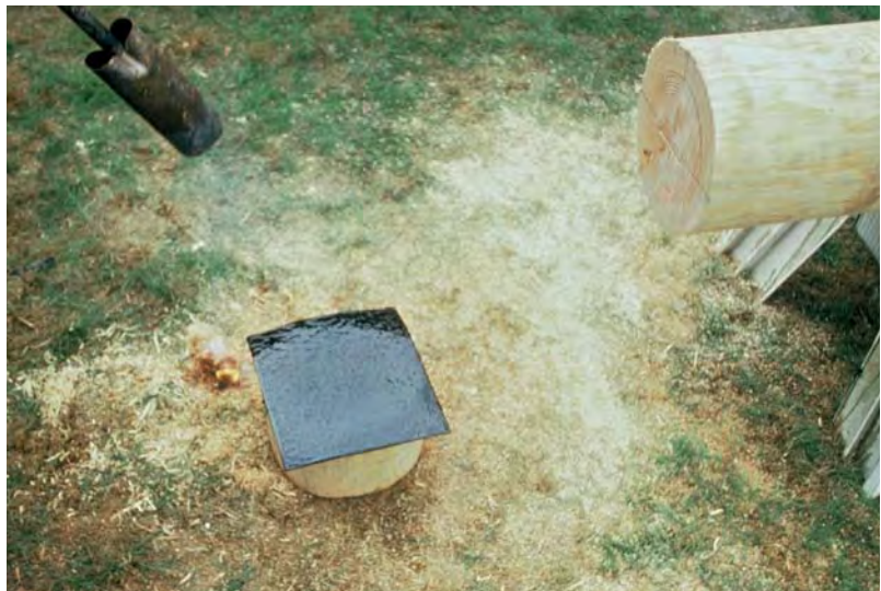
Figure 5. A propane-fired torch is used to heat torch-down roof membrane. Once heated, the membrane will be adhered to the bottom of the log post and trimmed to fit exactly. This membrane helps prevent water from wicking up the log and causing rot.
