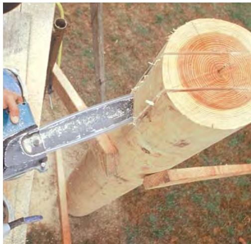
Figure 9. The pockets for beams also require plunge cutting with a chainsaw. The same safety rules apply, with the additional caveat that you should work from scaffolding for stability.
