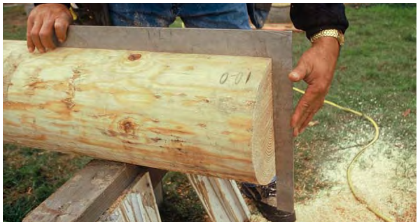
Figure 3. To mark the end of the log to be cut square to the centerline, a framing square is held to the layout line (left). It takes a little finesse to hold the pencil square to the square. After the cut, check for square (below), but remember to allow for any taper the log may have.
