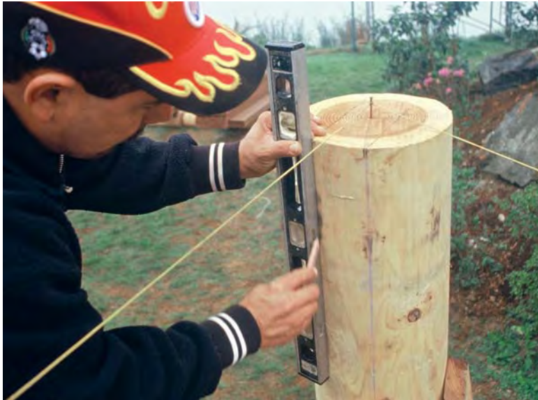
Figure 8. With the posts up and braced plumb, a string is used to establish the line of the beam. A carpenter uses a level to lay out the side cuts for the beam pocket.
