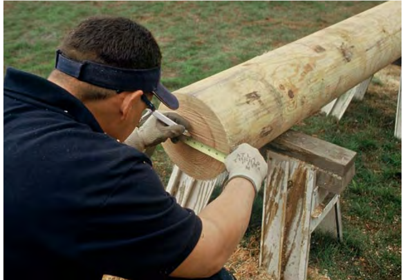
Figure 4. The hold-down anchor (above left) will fit in a slot cut in the post's bottom. The odds are that the anchor is not centered exactly on the pedestal. Measure carefully to ensure that the anchor slot is cut so that the post eventually will overhang the pedestal evenly.
