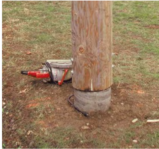
Figure 1. Log posts are vulnerable to rot from water wicking up the end grain. Sizing the portion of the footing that's above grade to be 2 inches smaller than the post provides a drip-edge. Keep the post at least 6 inches above grade to minimize the effect of rain splashing upward.
