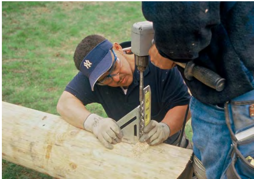
Figure 6. A torpedo level and a layout square are used to guide the drilling of holes for the bolts that will secure the log to the anchor.
