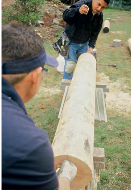
Figure 2. All layout on logs springs from a centerline. To find it, a plumb line is drawn through the center of each end of the log (far left); the points where these lines intersect the face of the log are joined with a chalk line (left).
