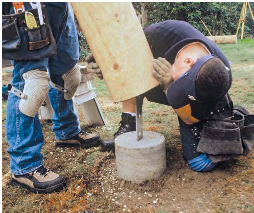
Figure 7. Placing the post is a two-person operation. Be sure the log is oriented correctly, and not 180 degrees off.
