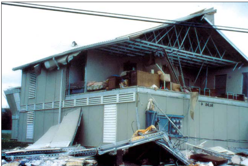
Once the gable end goes, it can unzip a house, not only devastating the structure but also ruining the entire contents of a home, which become saturated with water.
