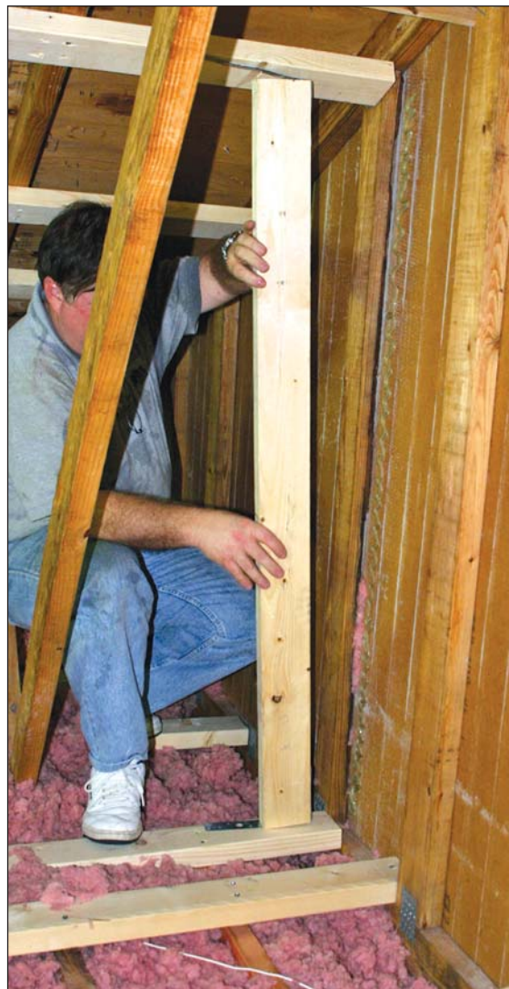
Assembling the pieces: After the horizontal braces get installed, metal straps must be preinstalled on the retrofit studs. These retrofit studs can then be installed by bedding them in a generous bead of an AFG-01-rated structural wood adhesive along the edge of each gable-end stud.
