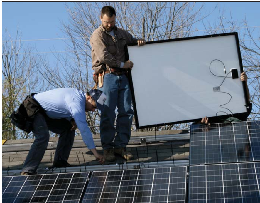
PLUG AND PLAY. These Kyocera PV panels are equipped with wires and plugs, allowing the panels to be connected in series as the array is mounted on the rooftop rails (left). Workers connect the plugs as they go (above). Connecting the entire array through the power inverter into the building's main electrical panel on the ground calls for a licensed electrician.
