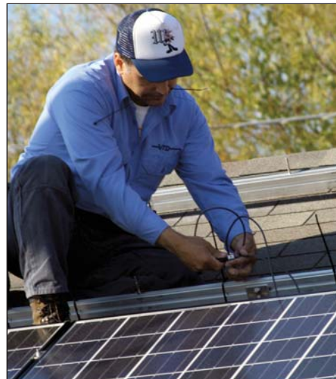
PLUG AND PLAY. These Kyocera PV panels are equipped with wires and plugs, allowing the panels to be connected in series as the array is mounted on the rooftop rails (left). Workers connect the plugs as they go (above). Connecting the entire array through the power inverter into the building's main electrical panel on the ground calls for a licensed electrician.
