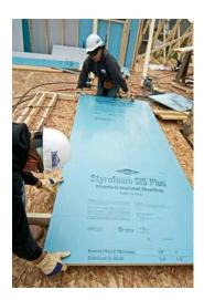
penetrations are properly sealed or flashed. Available in thicknesses of  $^{1}/_{2}$  inch (R-3.0) and 1 inch (R-5.5), panels come in 8-, 9-, and 10-foot lengths. The company says prices compare to those of OSB or plywood sheathing plus a separate WRB.
