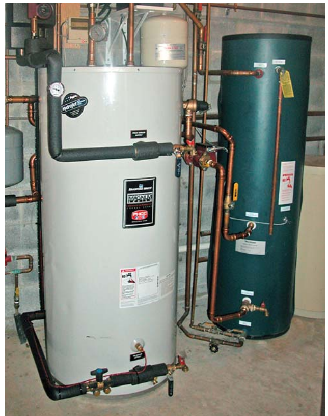
Figure 3. The author charges the closed solar loop that runs to the rooftop array with inhibited glycol, which keeps the system from freezing (above). The primary storage tank has a 120-gallon capacity, while the blue 75-gallon indirect tank supplies backup hot water on cloudy days (right).
