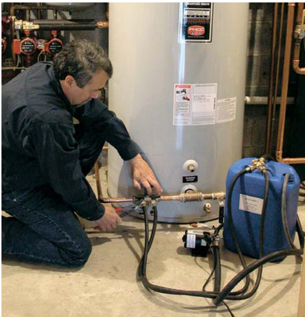
Figure 3. The author charges the closed solar loop that runs to the rooftop array with inhibited glycol, which keeps the system from freezing (above). The primary storage tank has a 120-gallon capacity, while the blue 75-gallon indirect tank supplies backup hot water on cloudy days (right).
