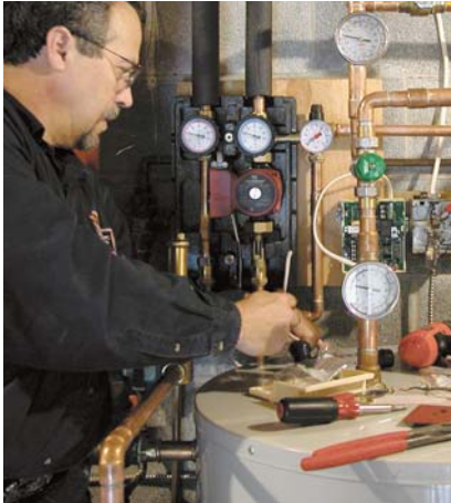
Figure 2. The system's circulation pump is part of a preassembled unit that also includes valves, gauges, and an air separator, which simplifies system design and installation.
